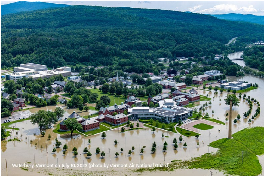
Figure 3: Waterbury Flooding at State Office Complex, July 10-11, 2023 (Vermont Air National Guard)
