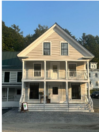
Figure 2: East Calais General Store, post rehabilitation
