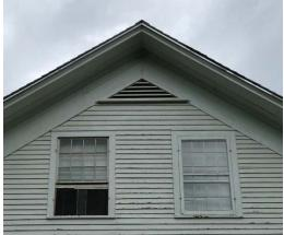
Gable vents allow air to circulate under the roof, drying trapped moisture. Courtesy of the Preservation Trust of Vermont.
