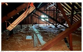
This loose fill cellulose may be mess, but it can easily be removed to allow for repairs and preservation of historic features.
