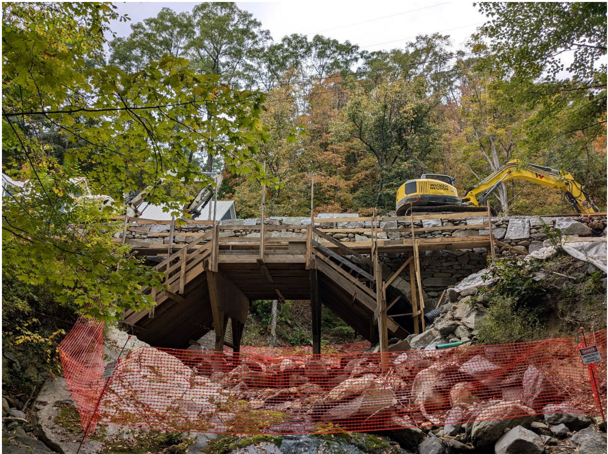
Figure 7: West Townshend Stone Arch Bridge Rehabilitation, September 2024
