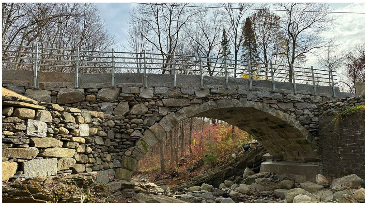
Completed Upstream View of Bridge and Wing Wall
