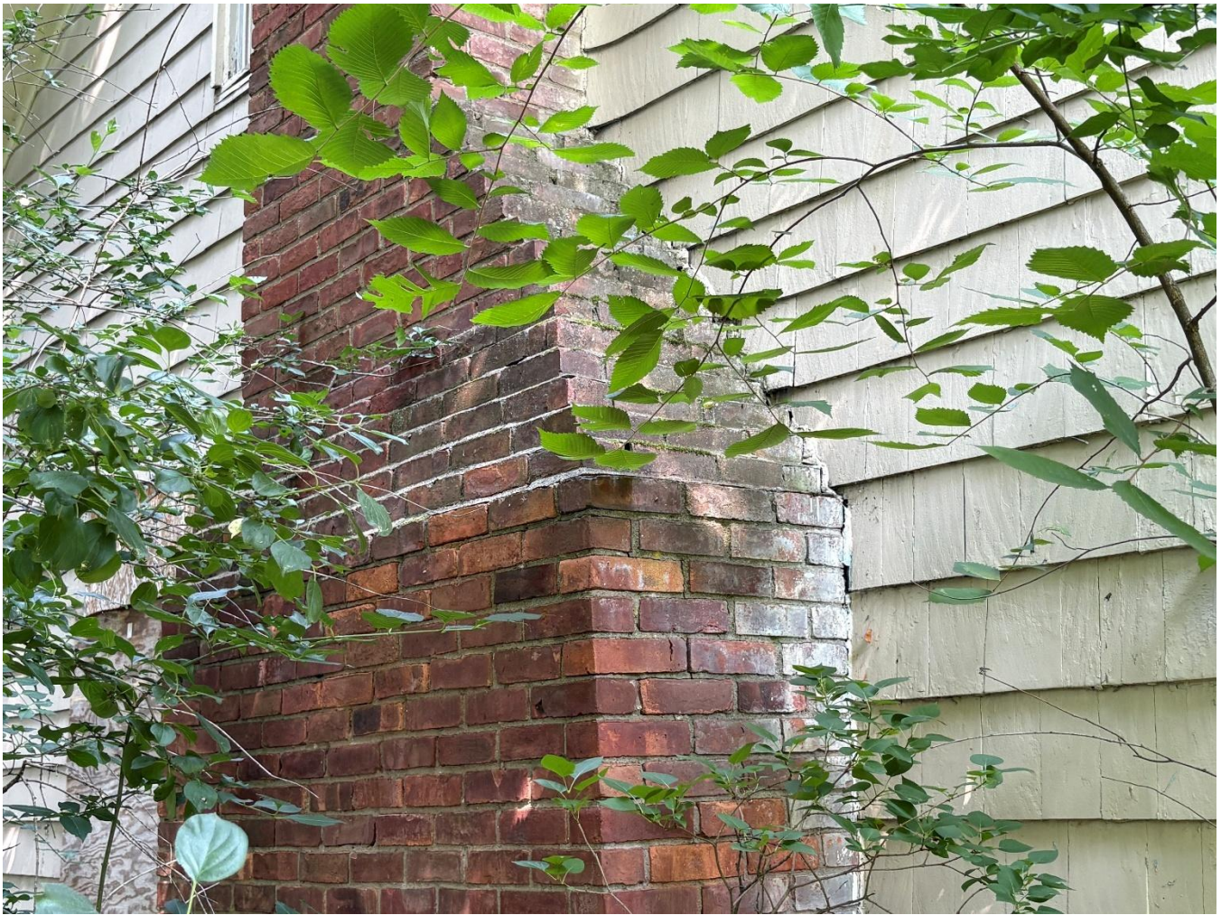
Image 11: Detail of exterior stepped chimney on south elevation.
