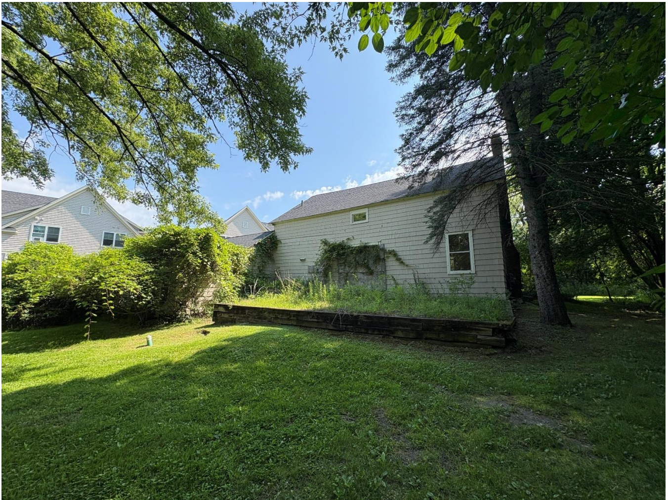
Image 8: Rear (west) elevation of the house.
