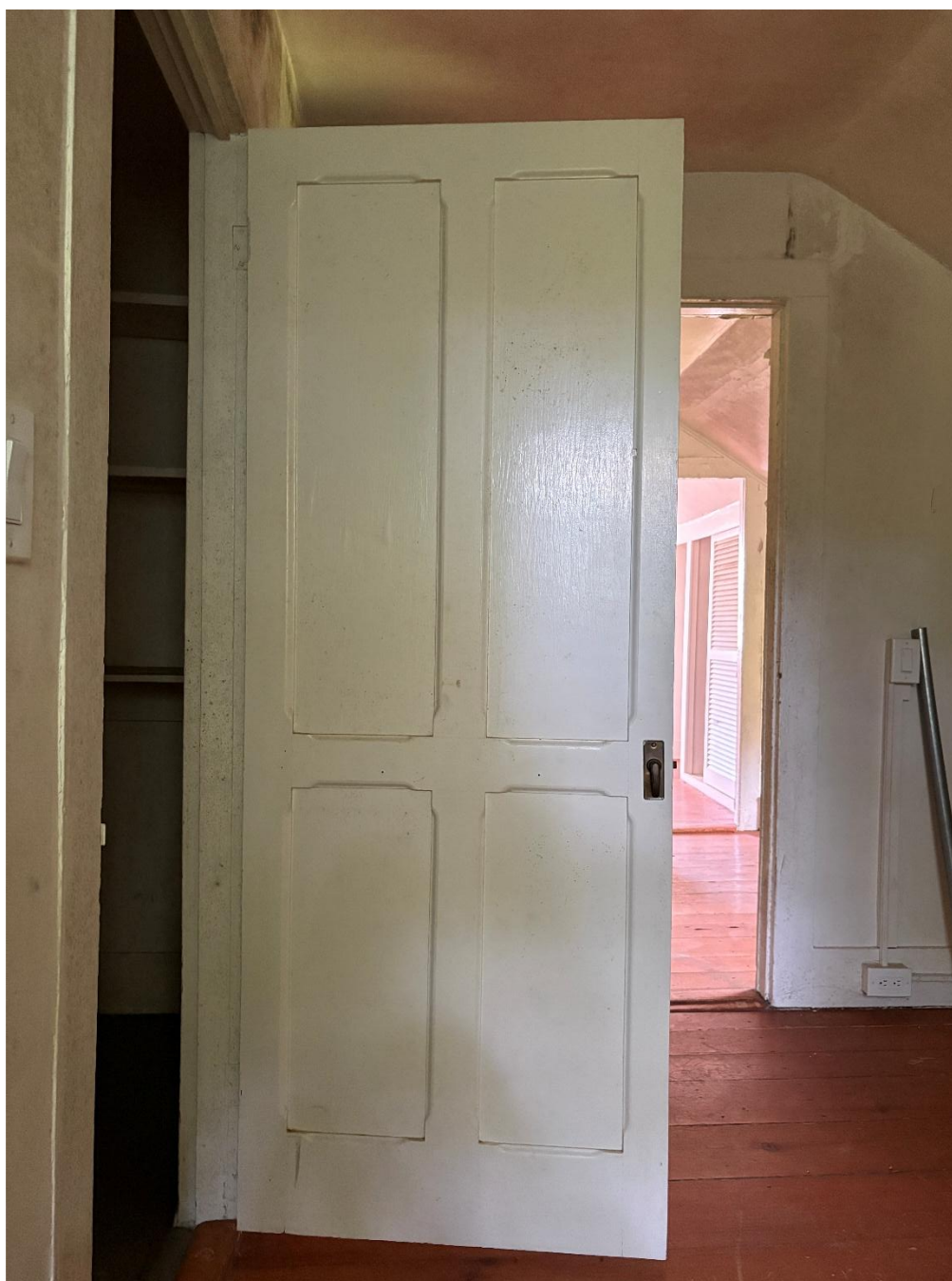
Image 31: Door details, southeast room, looking north.
