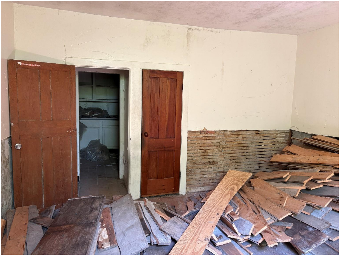
Image 17: View from northeast room, looking west to the passage and kitchen. A bathroom is behind the smaller door in the center.
