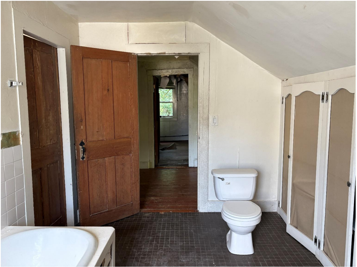
Image 28: Looking from the bathroom (northwest room) south to center hall and the southwest room. The door at left leads to another room.
