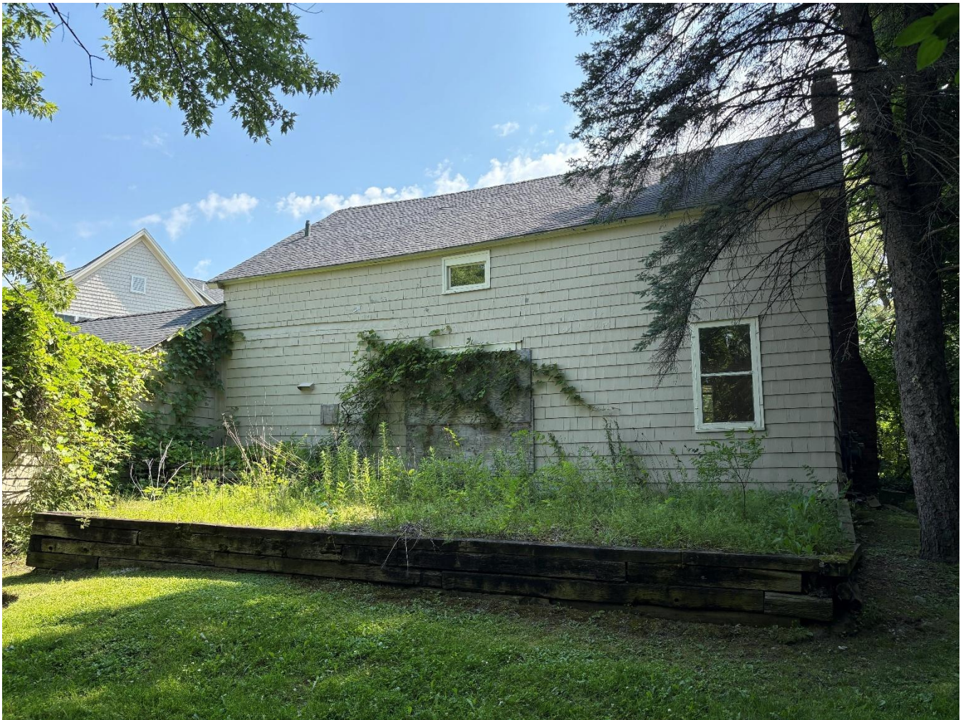
Image 9: Closer view of rear elevation shows an altered central bay.
