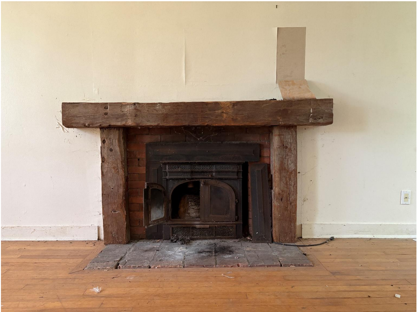
Image 21: Post and beam fireplace mantel on the southern wall of the southern room.
