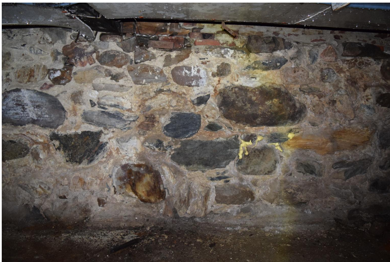
Image 36: Stone foundation wall, view from the basement staircase, looking east.
