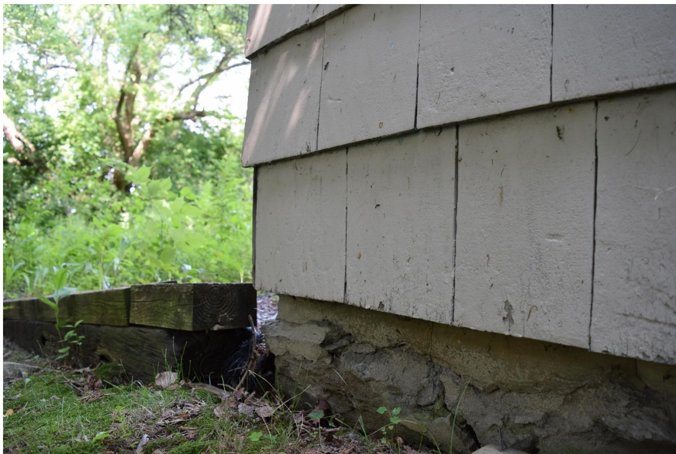
Image 12: Southwest corner of building shows wood shingle siding.
