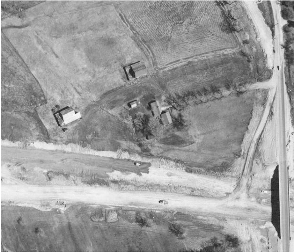
Figure 6: 1962 aerial image showing the house (center), large barns, and small outbuildings. By this time, the garage wing has been added. The construction of I-89 is underway, as seen in the bottom of the image. Source: VCGI.
