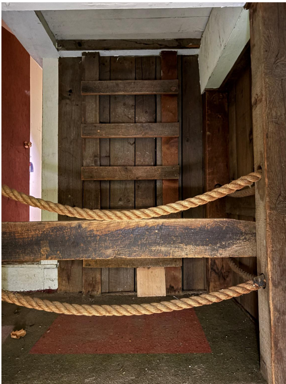
Image 42: A ladder provides storage access between the main house (see door at left) and the wing. Looking south.
