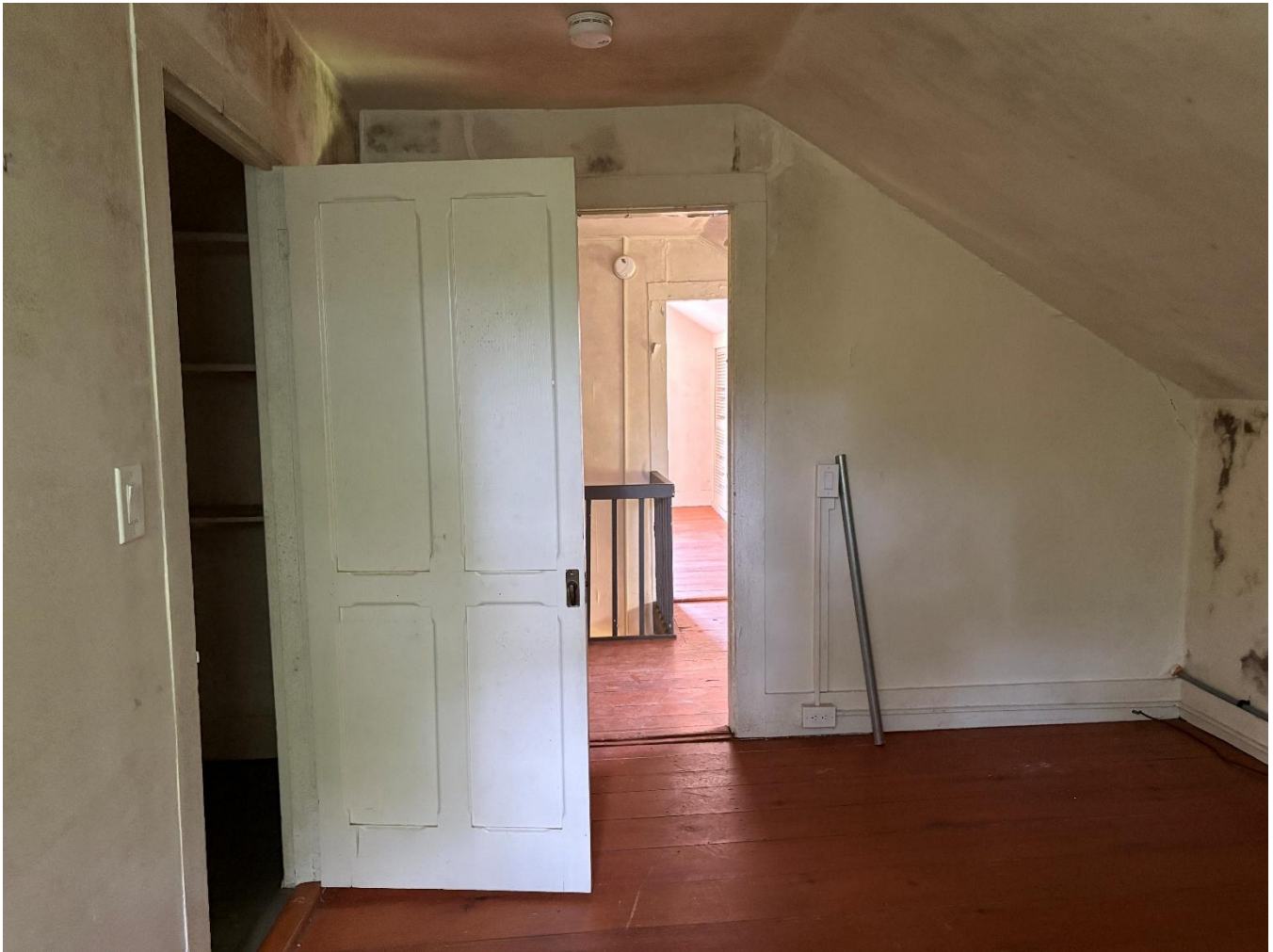
Image 30: View of the closet door in the southeast room. Looking north to the center hall.
