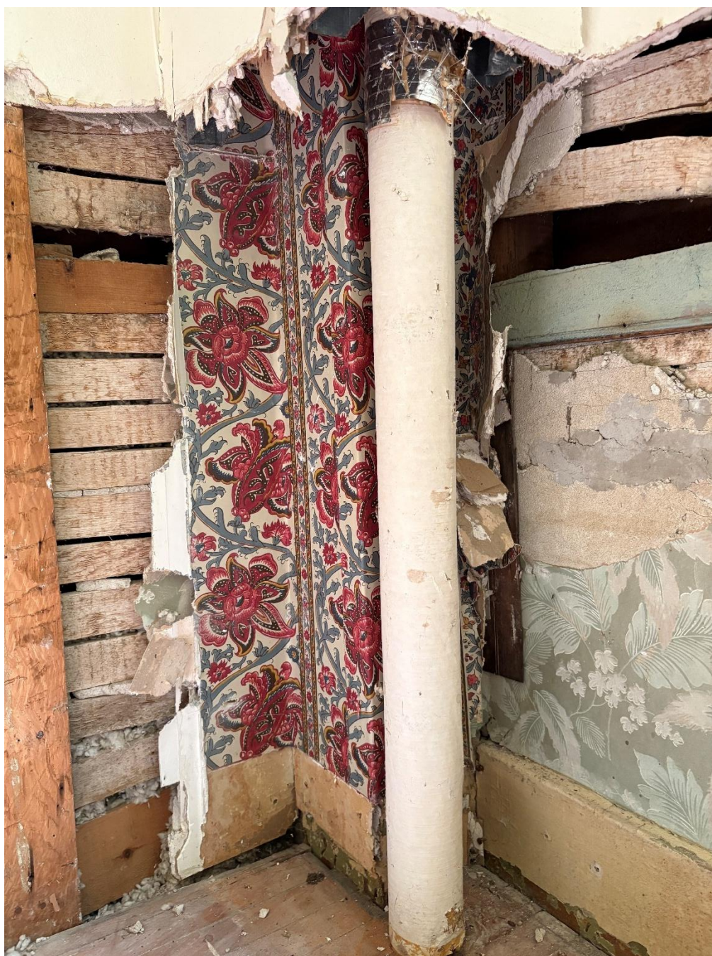
Image 16: Northeast corner of northeast room shows layers of wallpaper over plaster and lath.
