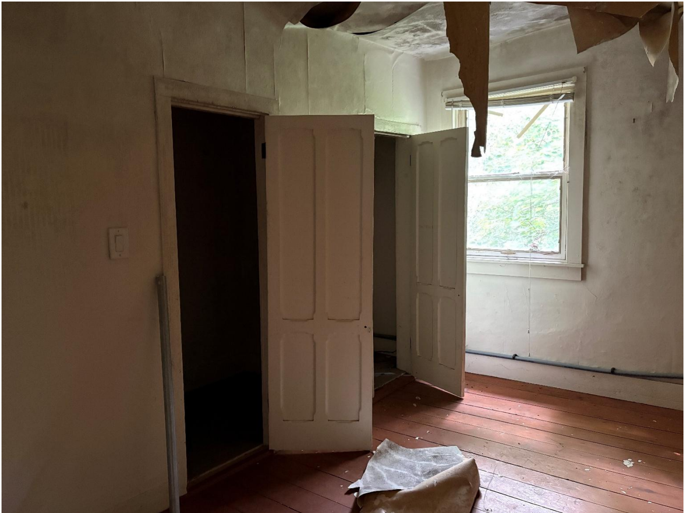
Image 26: Closet doors in the southwest upstairs room, looking southeast.
