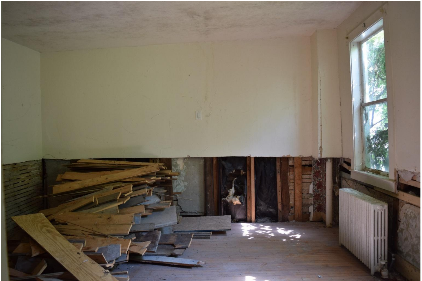
Image 15: Northeast front room, looking north. Partial walls have been removed as part of an abatement process.
