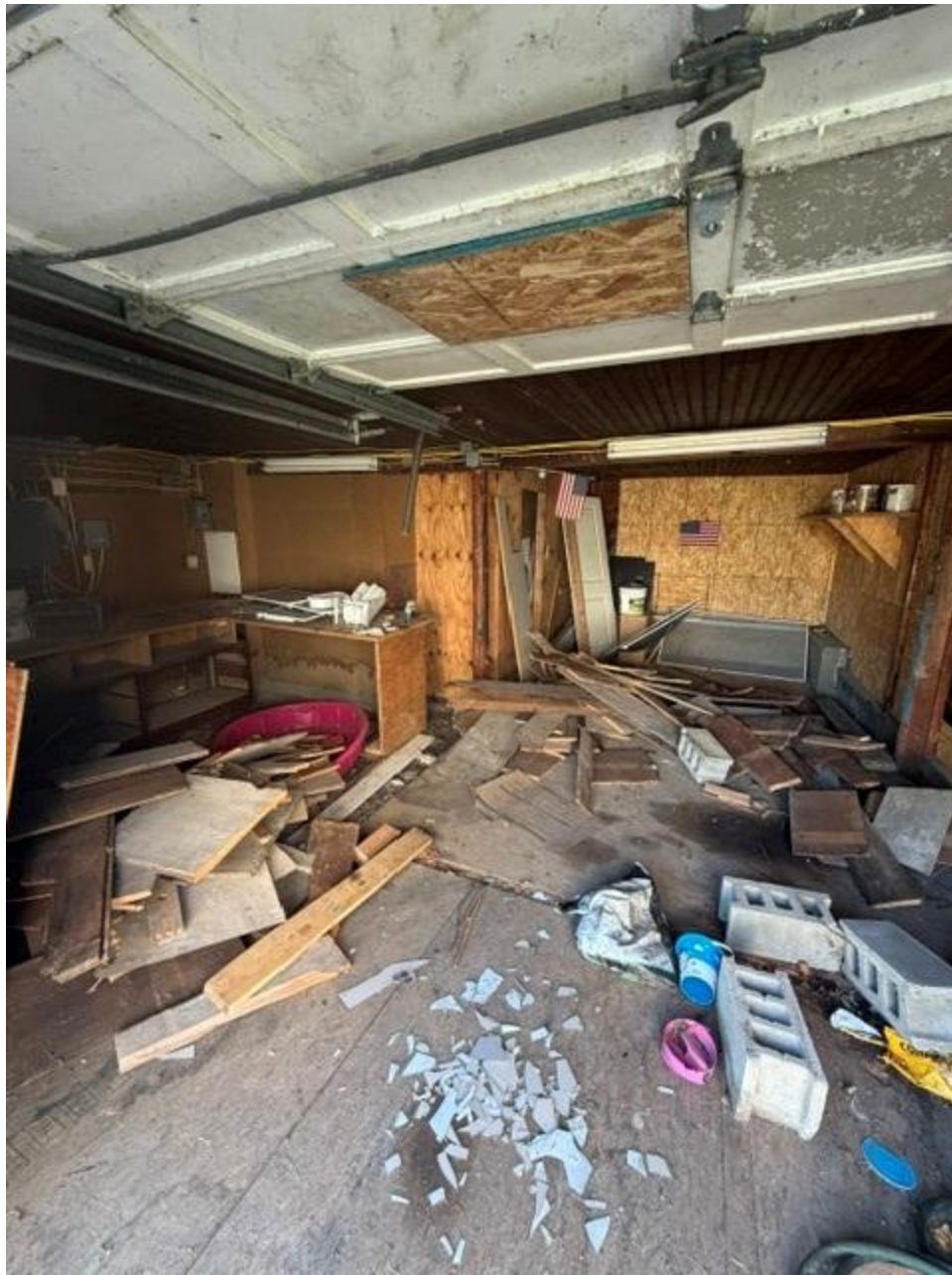
Image 44: Looking into the garage from the east garage door.
