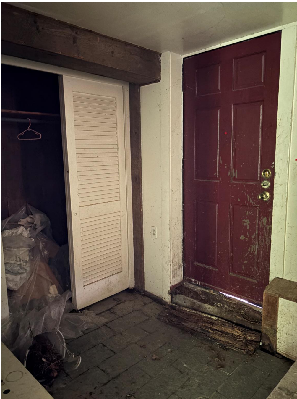
Image 40: Access to the wing is from the east façade of the garage wing.
