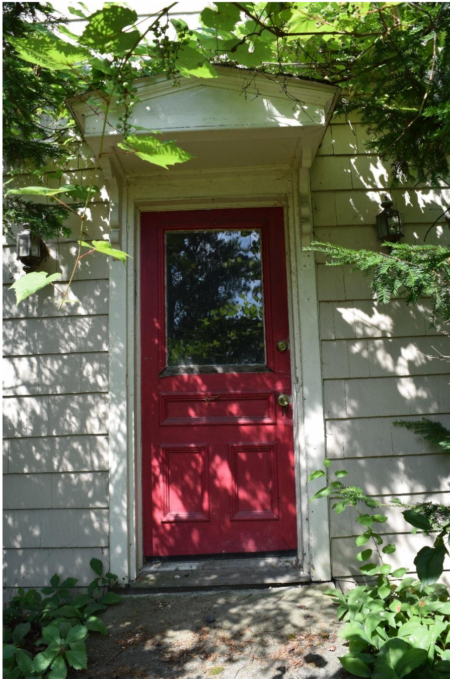
Image 4: Central façade entrance.
