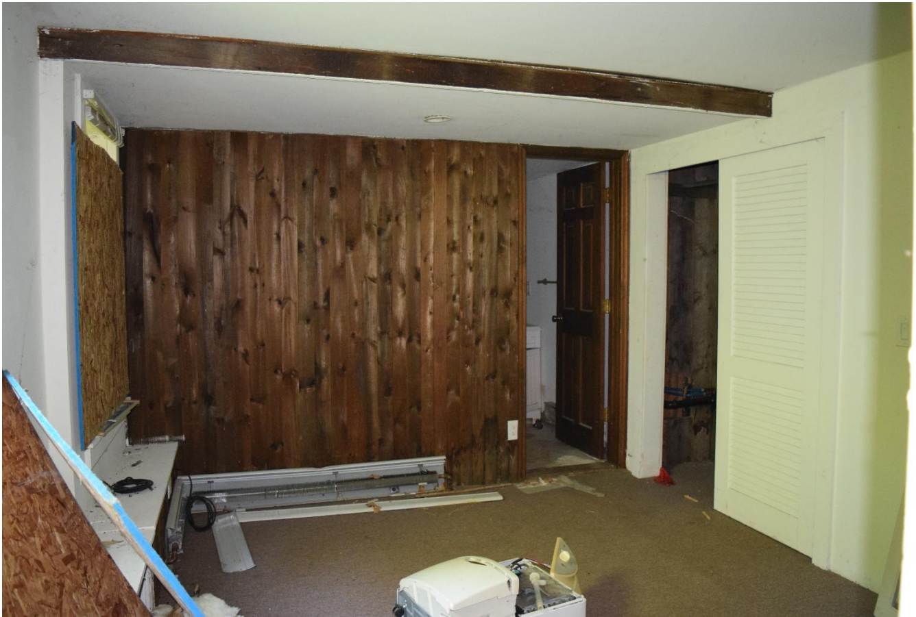
Image 39: Bedroom in the wing, looking north. Behind this room is the bathroom. A closet is at right.
