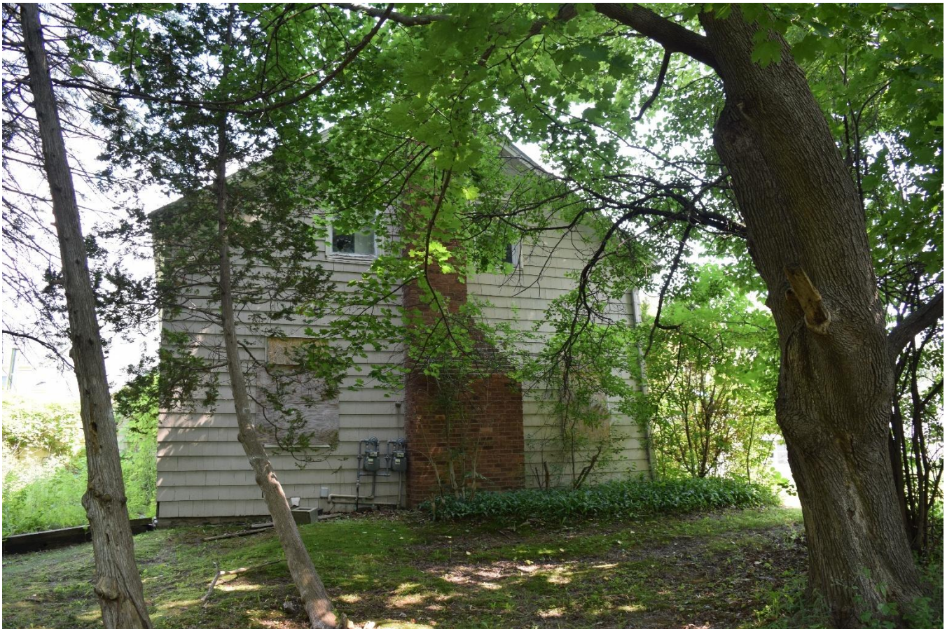
Image 10: South elevation with stepped chimney.
