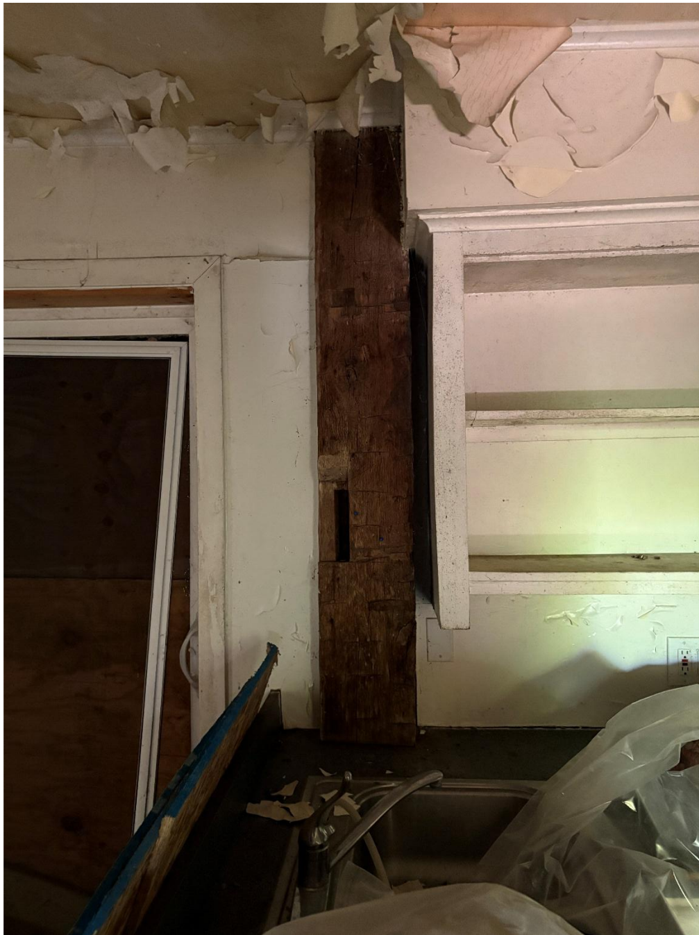
Image 19: View of post and beam framing in the kitchen, indicating this space has been opened up. A rear door is seen at left – a sliding door. It is covered with plywood on the exterior.
