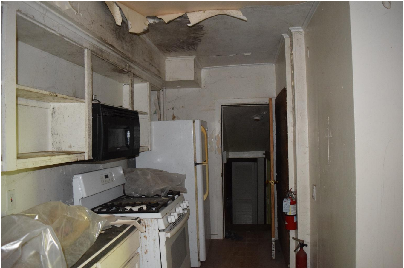
Image 18: View looking north through the kitchen to the wing. The kitchen is the northwest room of the house.
