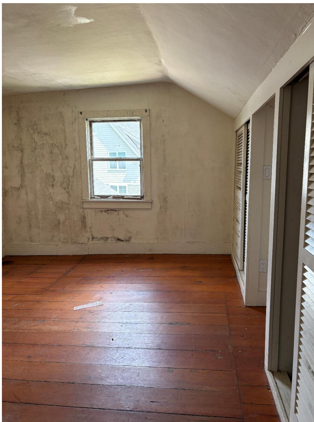
Image 34: Northeast upstairs room, looking north.
