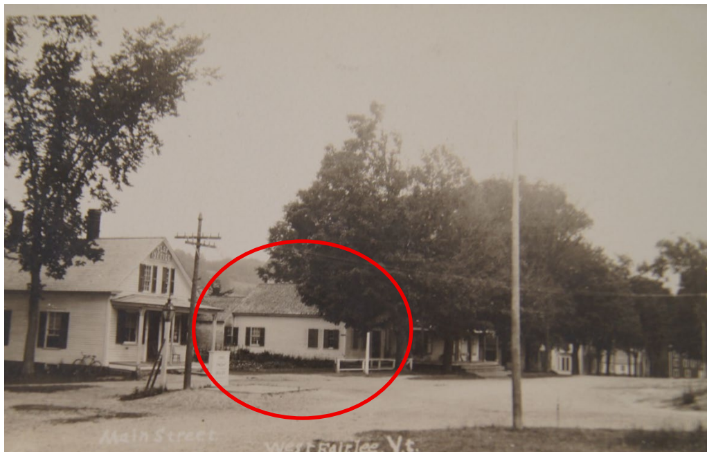
Resource No. 15 Historic Period Photograph No. 2: C. 1909 View Prior to Second Story. UVM Landscape Change Program, C. Abbott Collection.
