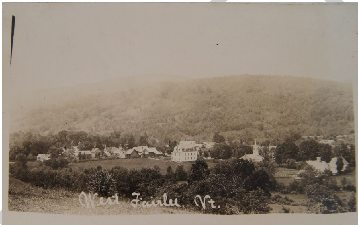
Figure 24: Looking southwest across West Fairlee Village from pastured hillside, note Bean Hall (Contributing Resource No. 38) and the West Fairlee Congregational Church (Contributing Resource No. 41) as well as the residential development along Mill Street, c. 1920 (West Fairlee Historical Society)
