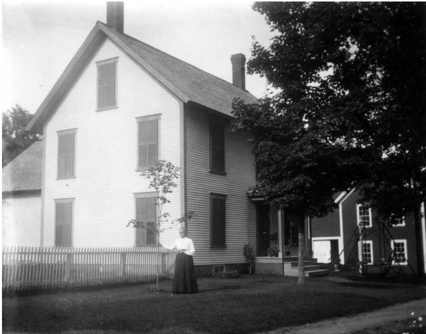
Resource No. 28 Historic Period Photograph No. 1: C. 1880 View with Carriage Manufactory, Since Removed, in Background. UVM Landscape Change Program, C. Abbott Collection.
