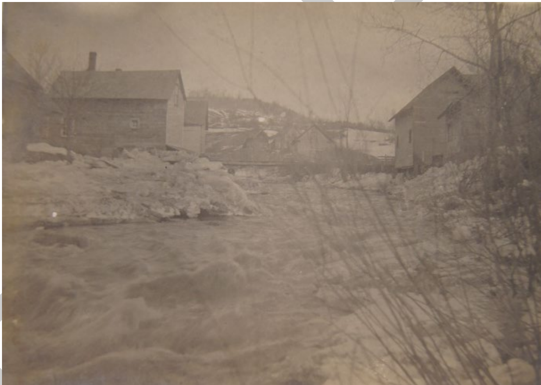
Figure 27: Looking north up the Ompompanoosuc River toward Mill Street, mills flanking, c. 1910s. No longer extant and burned in 1921. (West Fairlee Historical Society)
