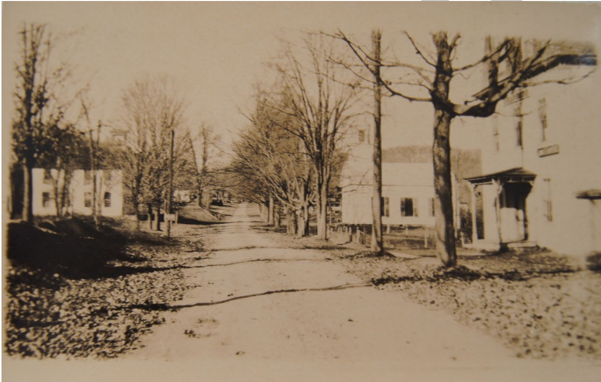
Figure 20: Looking north on Vermont Route 113/ Main Street. Bean Hall, Contributing Resource No. 38, and West Fairlee Congregational Church, Contributing Resource No. 41, line east side of road. Former West Fairlee Village School at right, no longer extant, c. 1905. (West Fairlee Historical Society)
