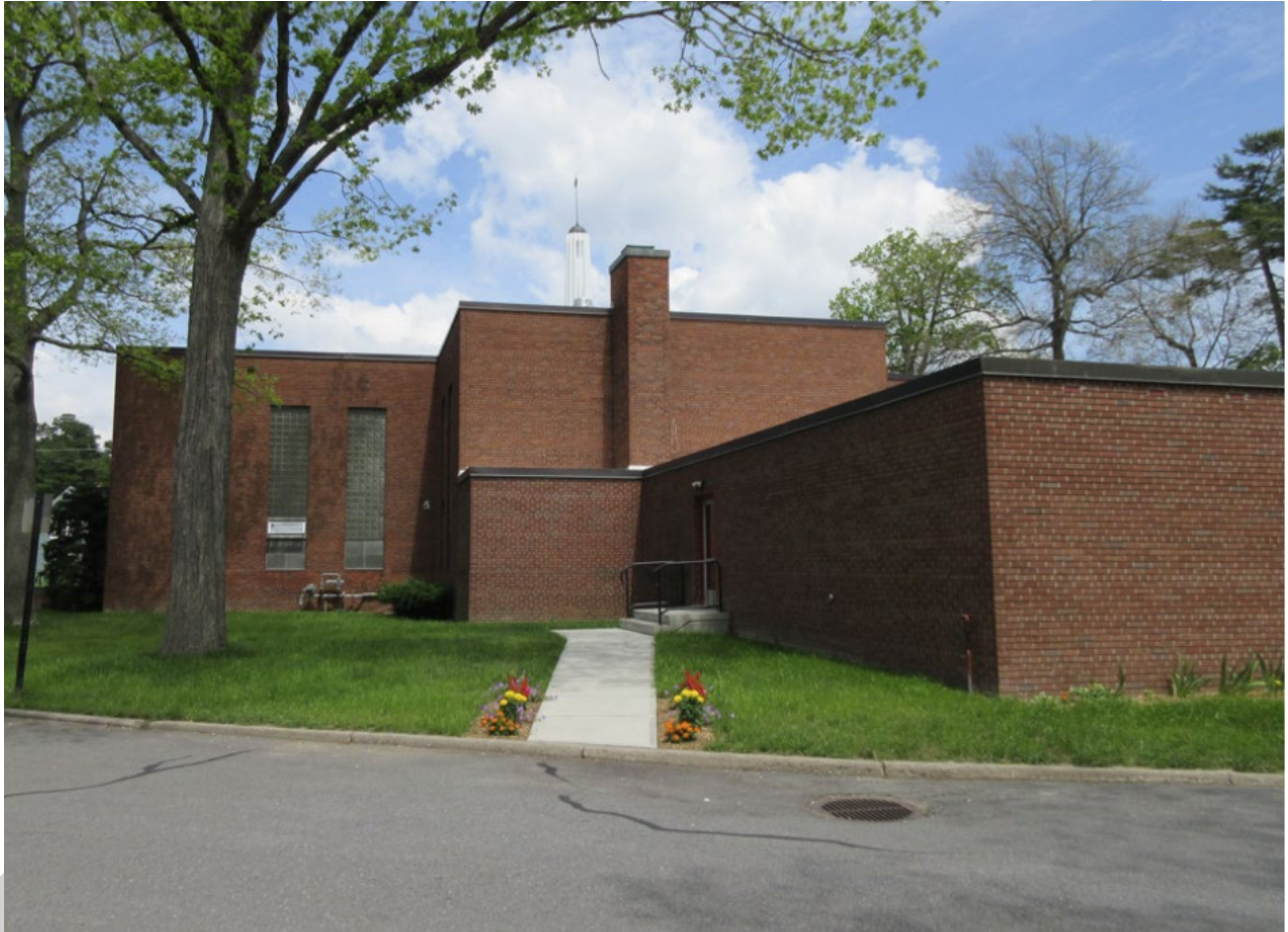
Figure 6: St. Mark's Church in Burlington, Vermont was indicative of a growing modern face in Catholic architecture. The church was constructed in 1941 and designed by Architects Freeman French Freeman.
