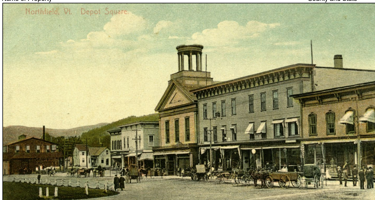
Figure 20: Circa 1915 postcard showing the north side of Depot Square. From right to left, 14 Depot Square (Extant), the Central Block (nonextant), the Universalist Church (extant), 29-35 Depot Square (nonextant), and 37-43 Depot Square (nonextant) are visible. Image courtesy of Norwich University Archives. 84
