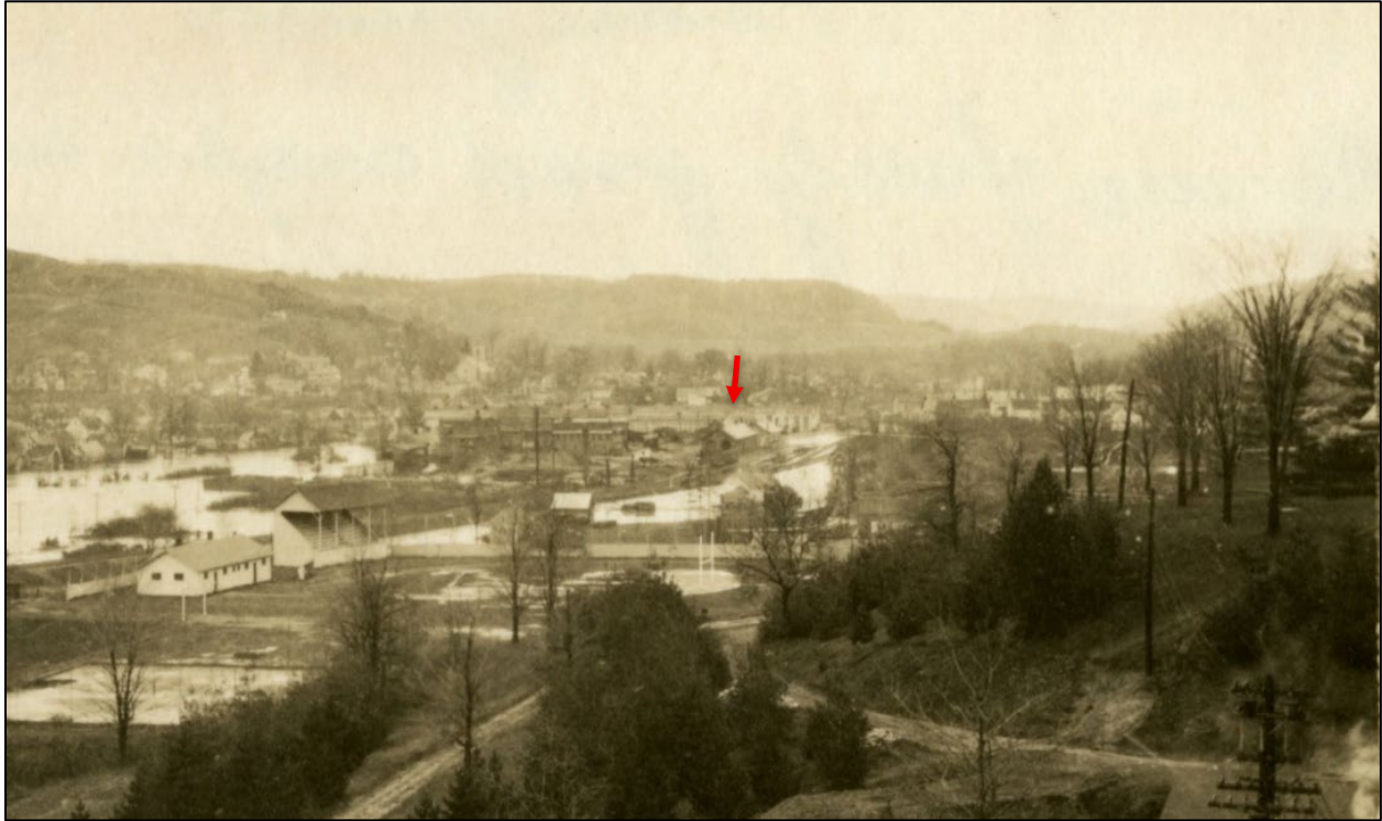
Figure 24: Photograph from November 1927 showing the immediate aftermath of the flood of 1927. In the photograph, floodwaters have inundated the former railyard and Water Street. Many of the buildings within the historic district were not damaged by the floodwaters. The Vermont Central Railroad Engine House is visible near the center of the image. It is denoted by a red arrow. Image courtesy of Norwich University Archives. 86
