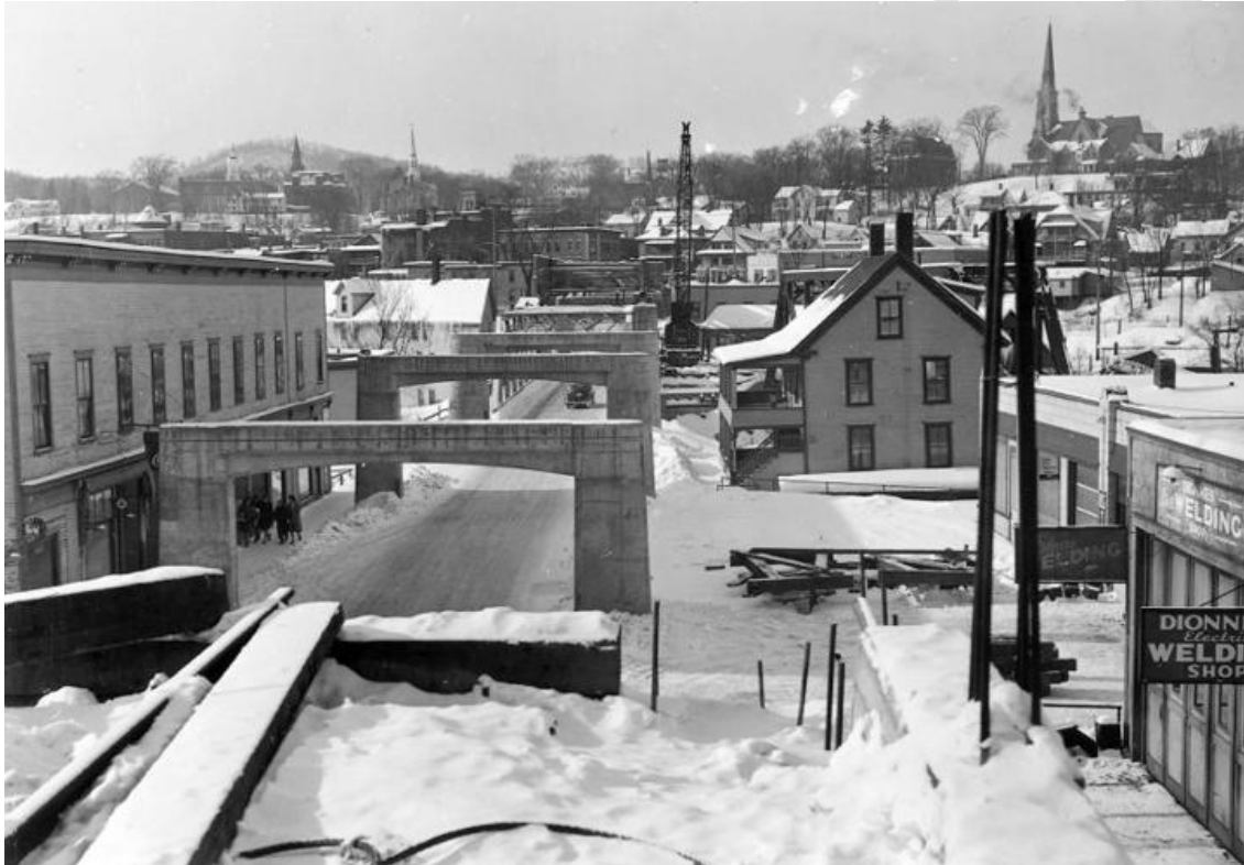
Figure 12: In 1943, the completion of the Portland Street Overpass cemented Portland Street as an increasingly auto-centric corridor, with the overpass eliminating the bottlenecks of the at-grade crossing and introducing an increasingly industrial and commercial sensibility to the corridor as it extended from Railroad Street. Photograph courtesy of the St. Johnsbury History and Heritage Center.
