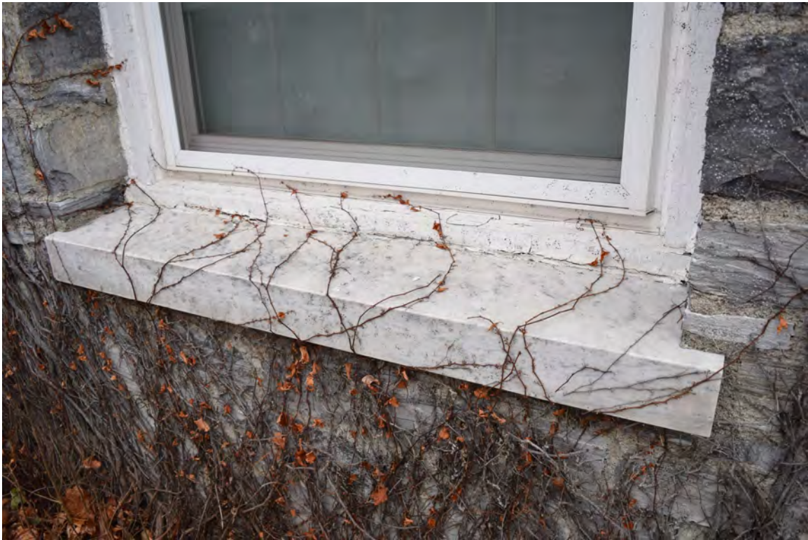
Photo 45: View shows typical marble window sill detail
