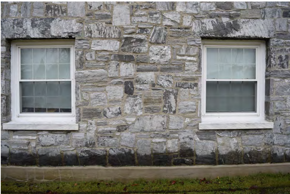
Photo 28: Looking south, view shows concrete foundation, limestone cladding detail on north section lower wall, and replacement vinyl windows
