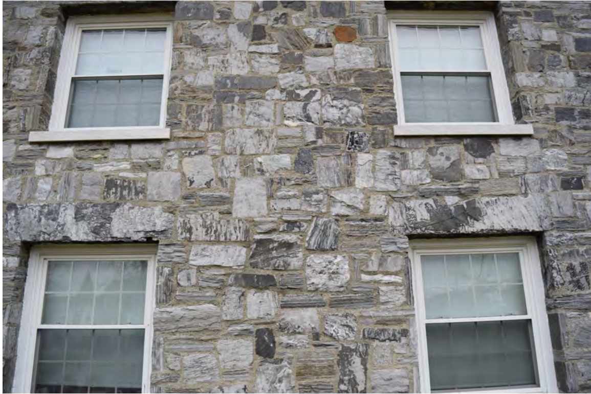
Photo 27: Looking south, view shows limestone cladding detail on north section upper wall and replacement vinyl windows
