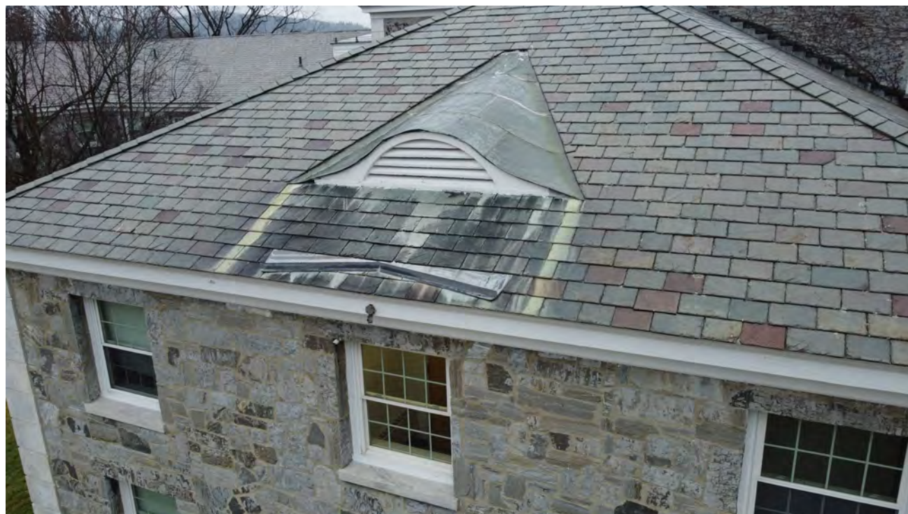
Photo 06: Looking northeast, view shows eyebrow dormer on west hip of center section
