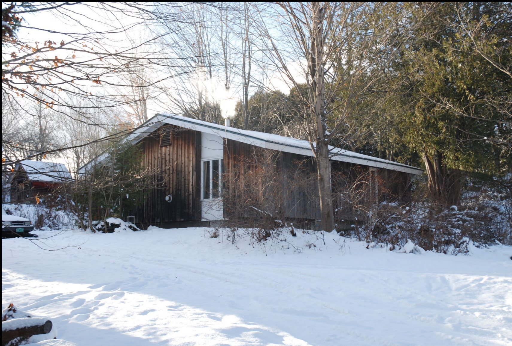
VT_Washington County_Maple Corner_018
