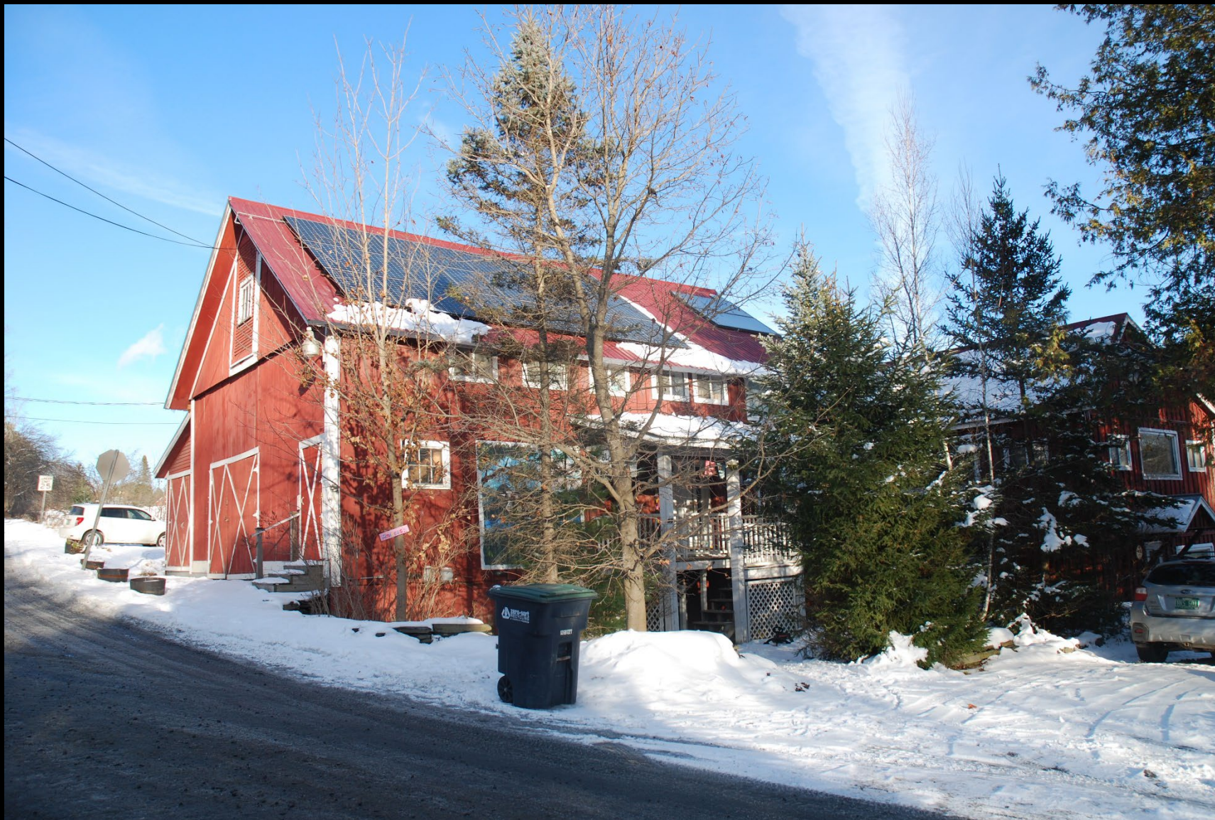
VT_Washington County_Maple Corner_006
