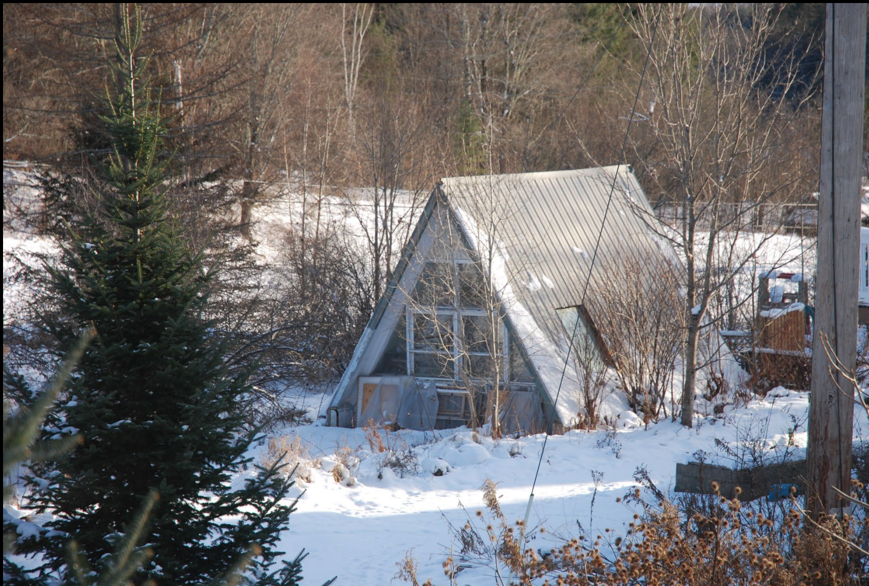
VT_Washington County_Maple Corner_007
