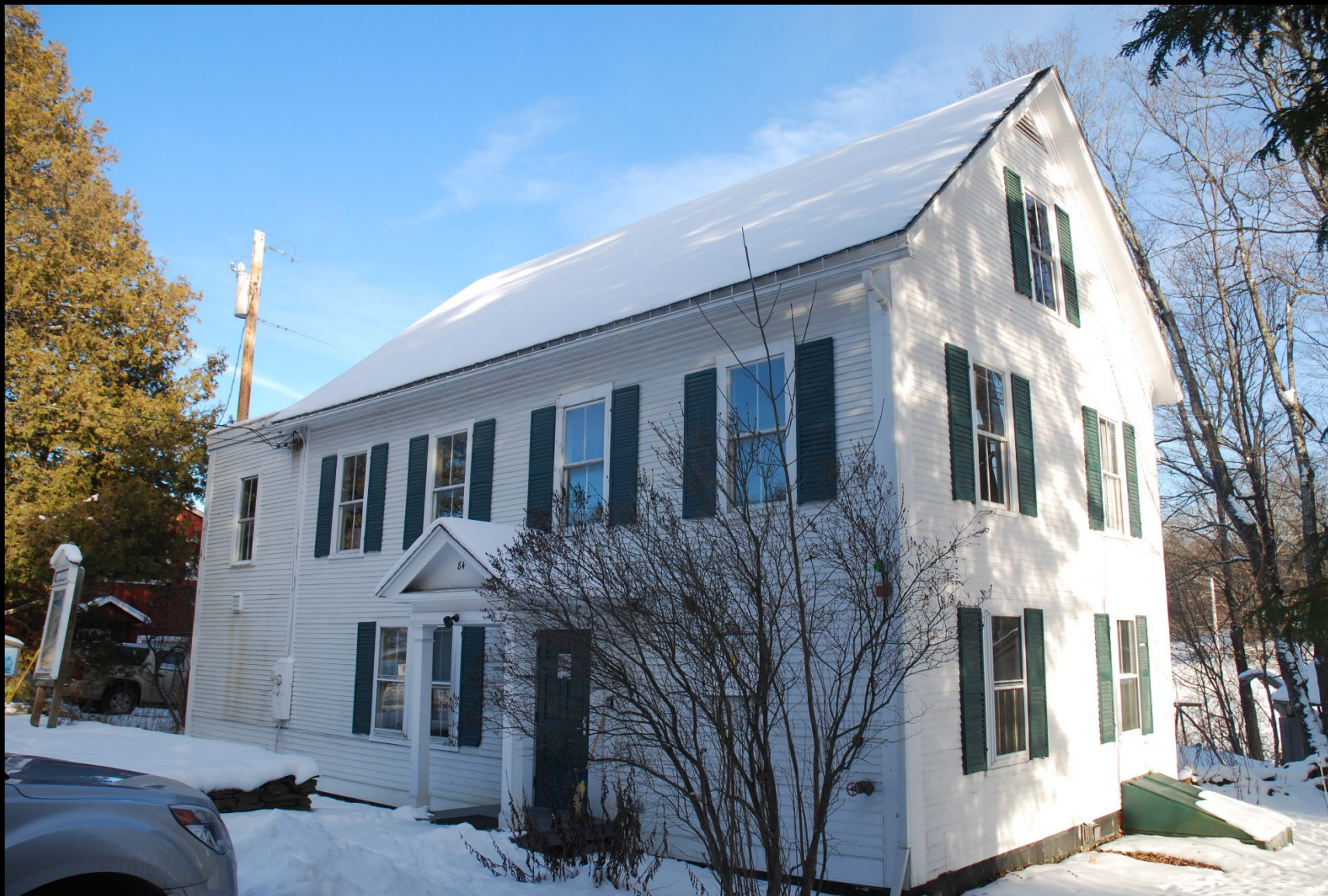
VT_Washington County_Maple Corner_008
