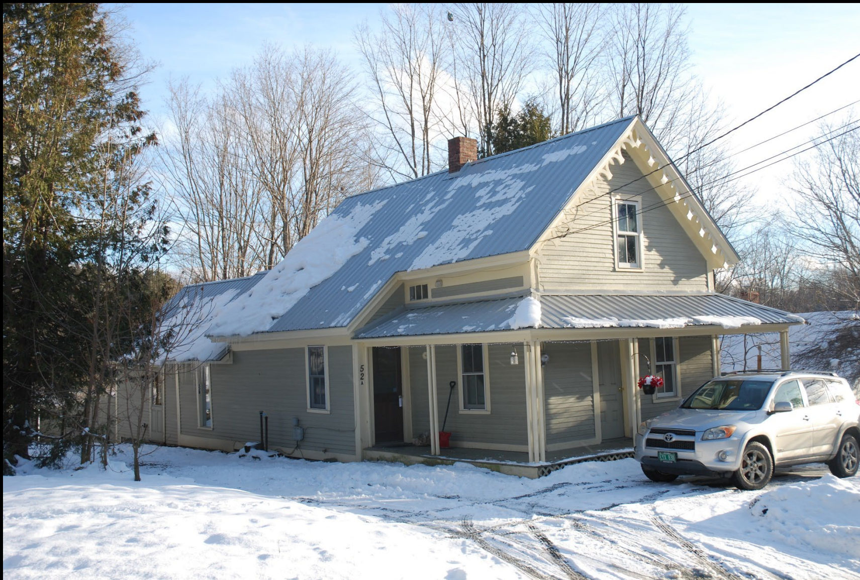
VT_Washington County_Maple Corner_011
