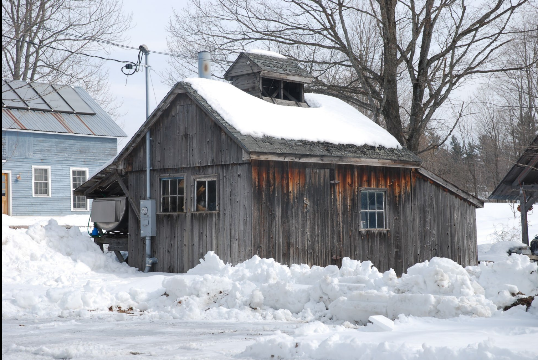
VT_Washington County_Maple Corner_003
