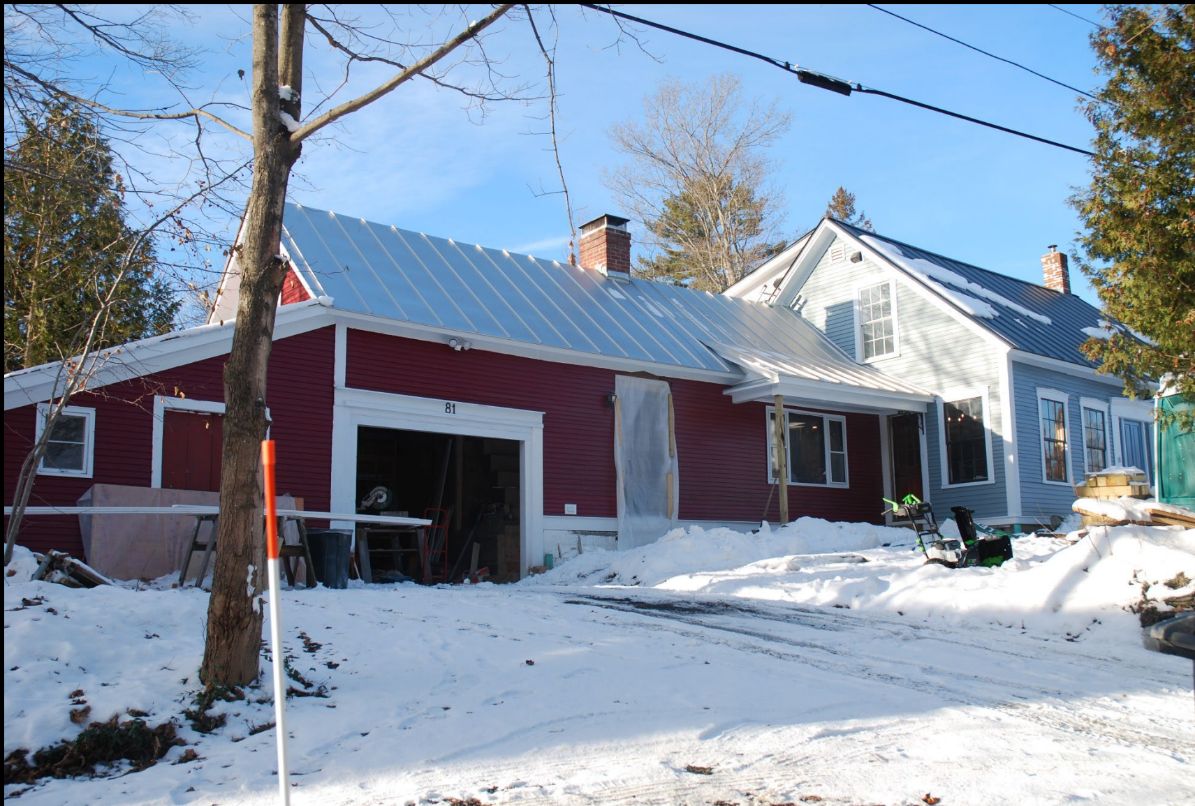
VT_Washington County_Maple Corner_029
