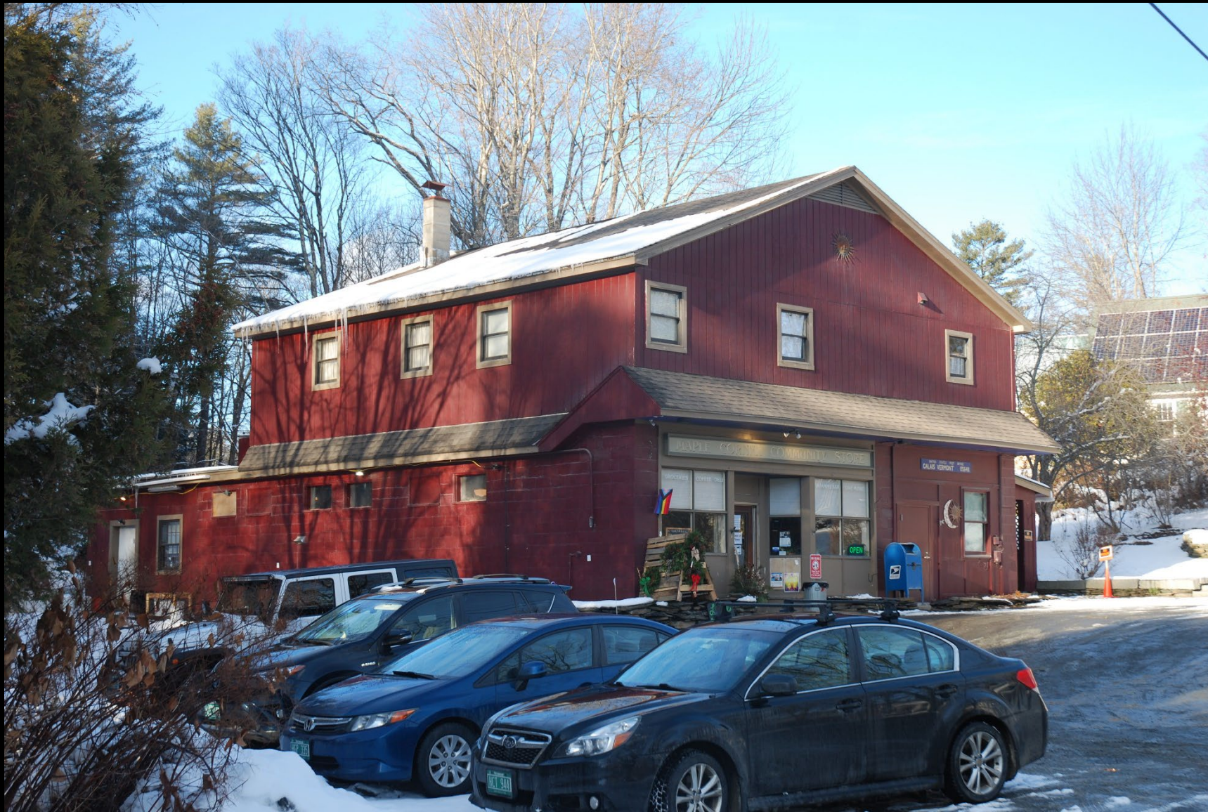
VT_Washington County_Maple Corner_025
