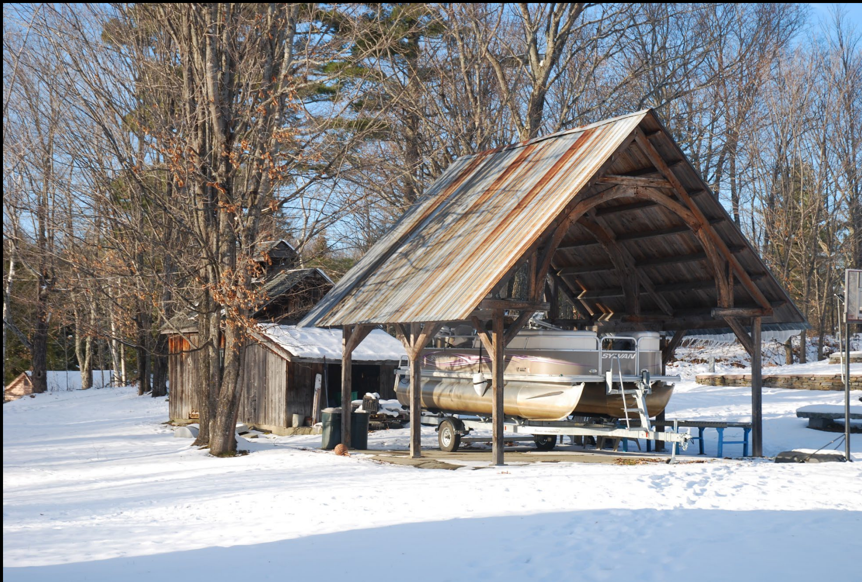
VT_Washington County_Maple Corner_005
