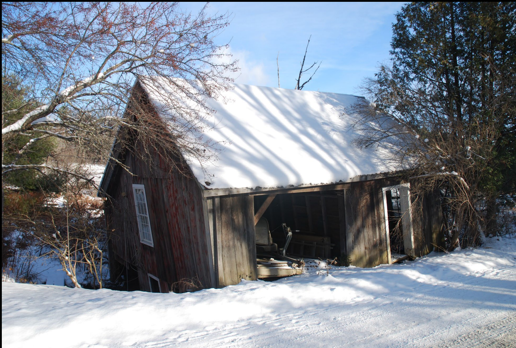
VT_Washington County_Maple Corner_015
