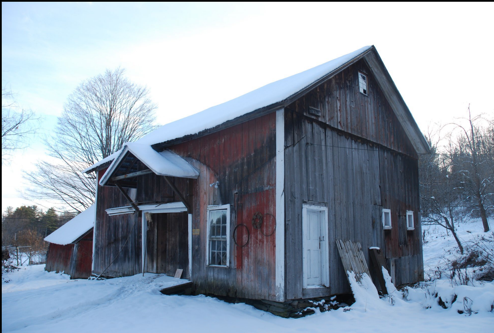
VT_Washington County_Maple Corner_019
