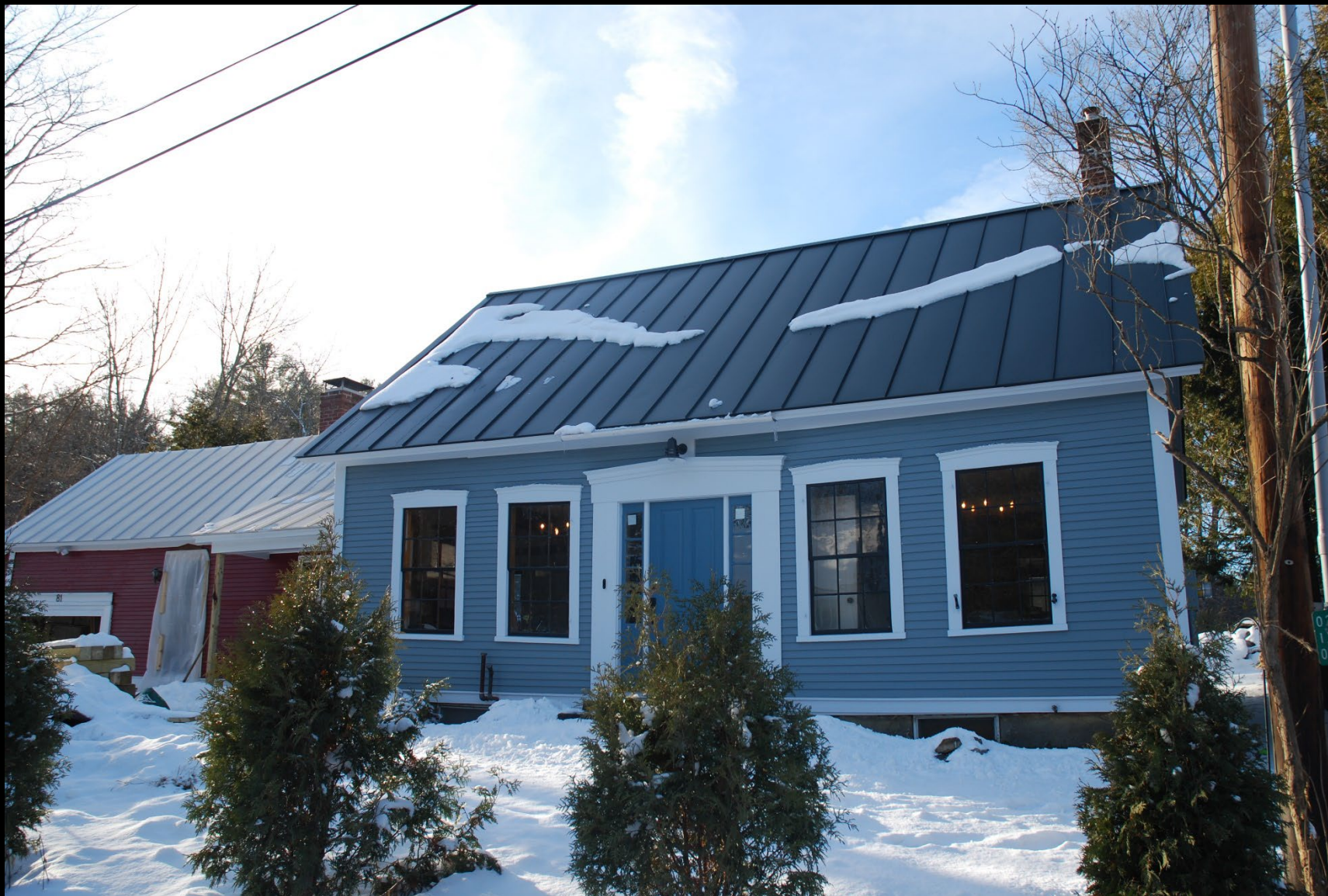
VT_Washington County_Maple Corner_030
