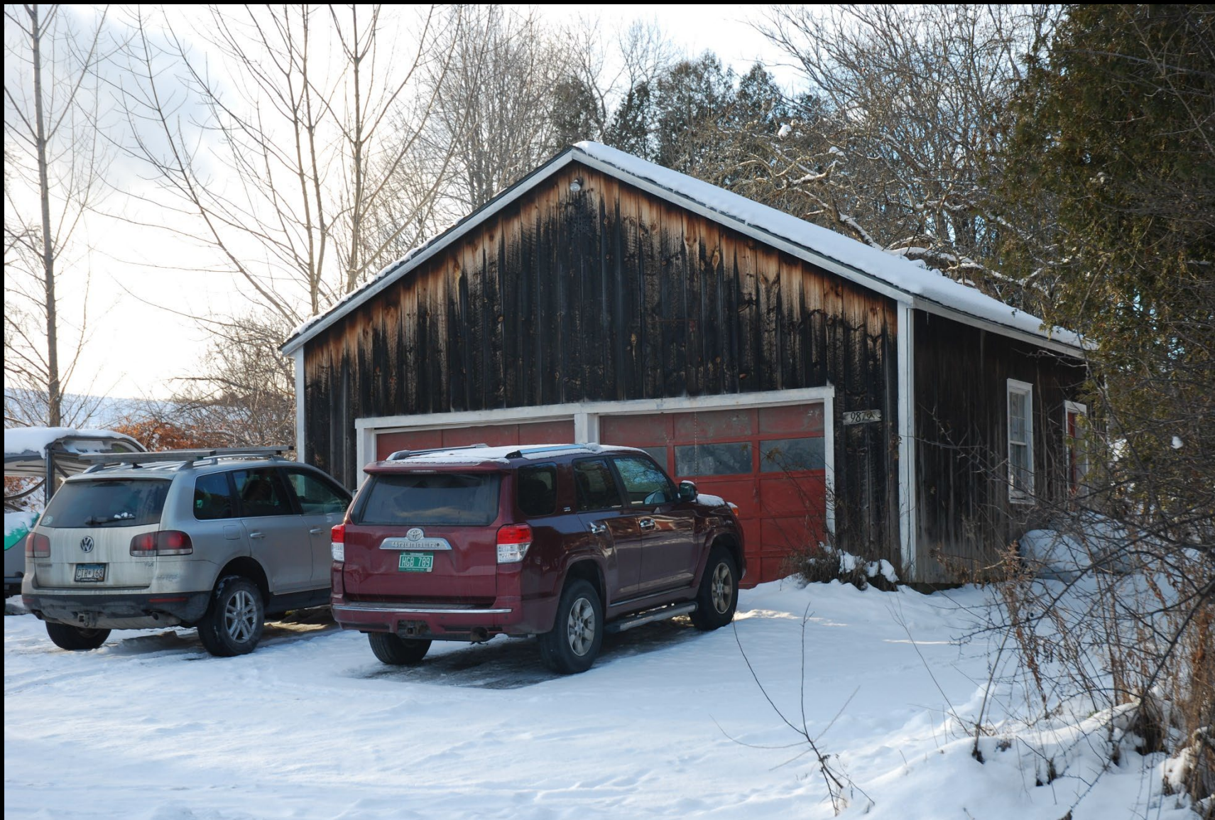
VT_Washington County_Maple Corner_023
