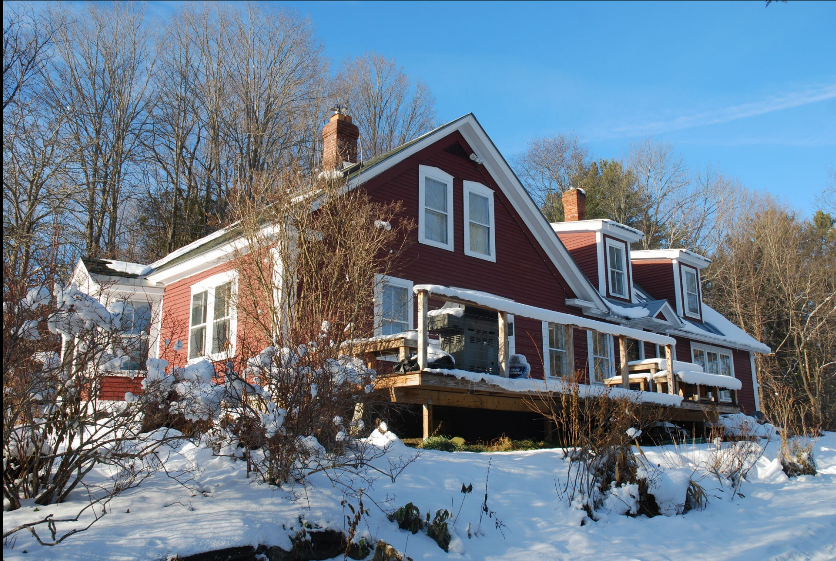
VT_Washington County_Maple Corner_022
