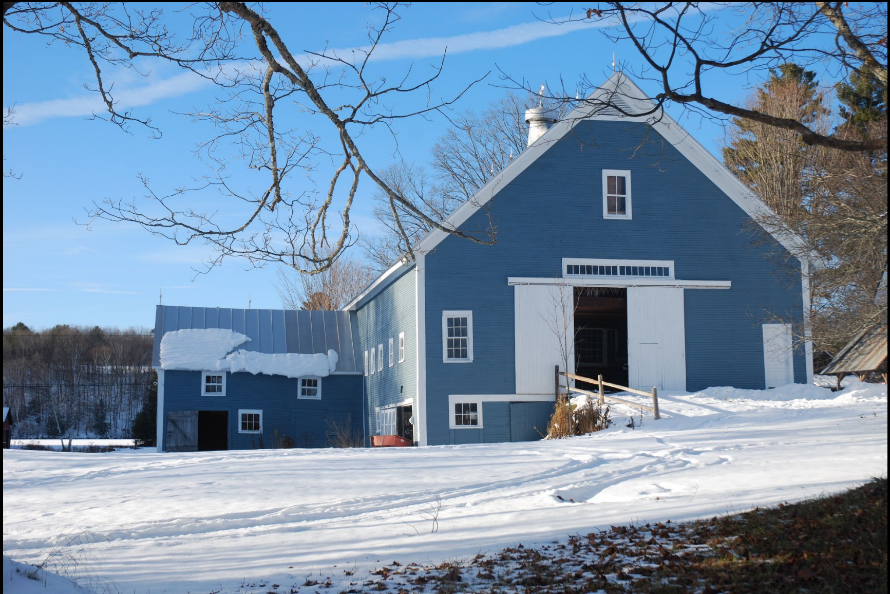
VT_Washington County_Maple Corner_002
