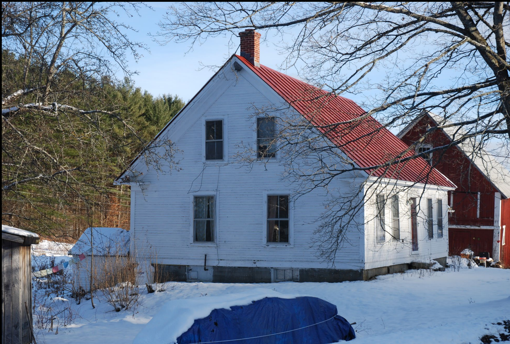
VT_Washington County_Maple Corner_016
