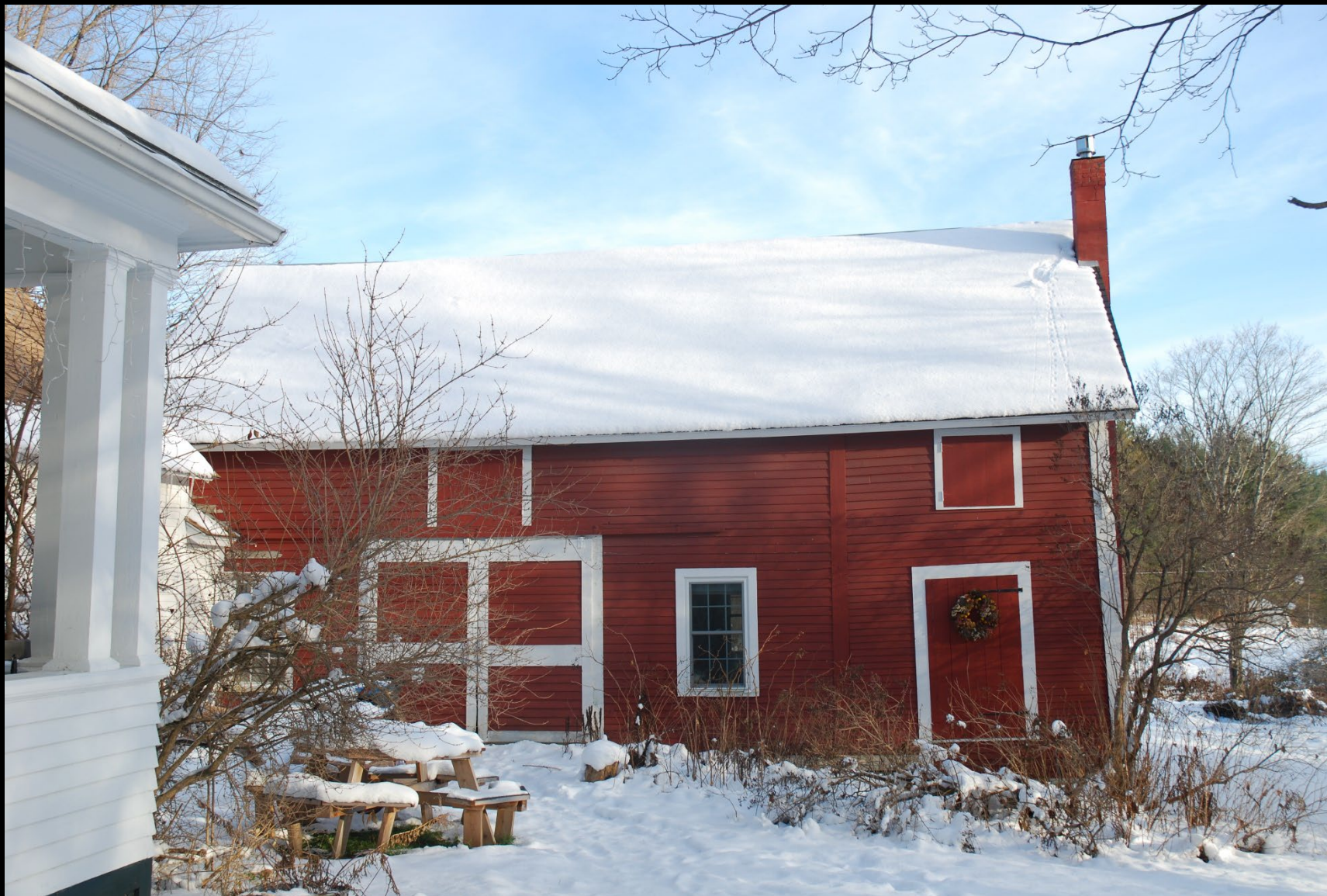
VT_Washington County_Maple Corner_013
