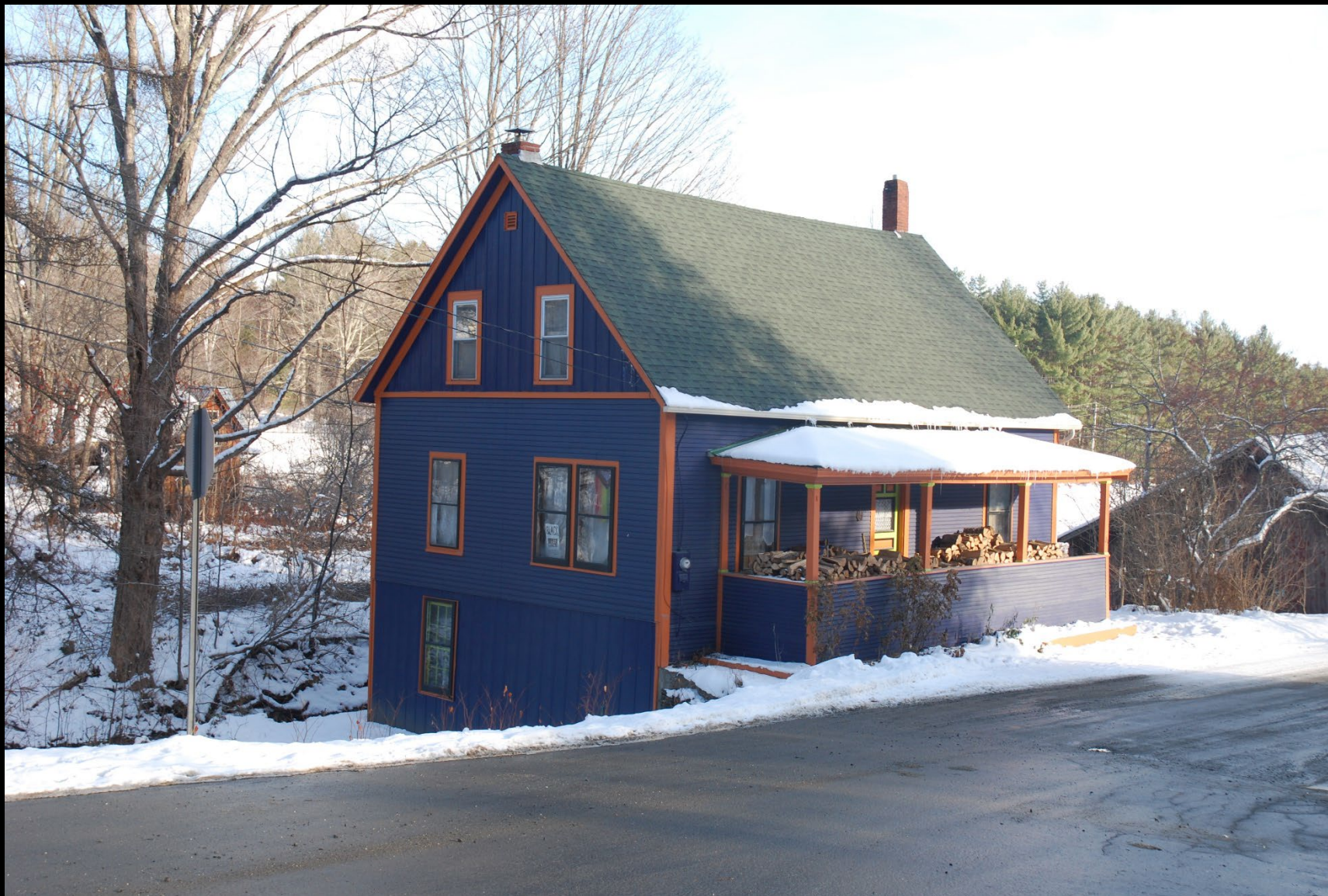
VT_Washington County_Maple Corner_014
