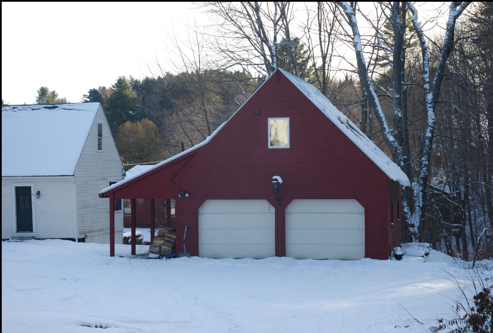
VT_Washington County_Maple Corner_028
