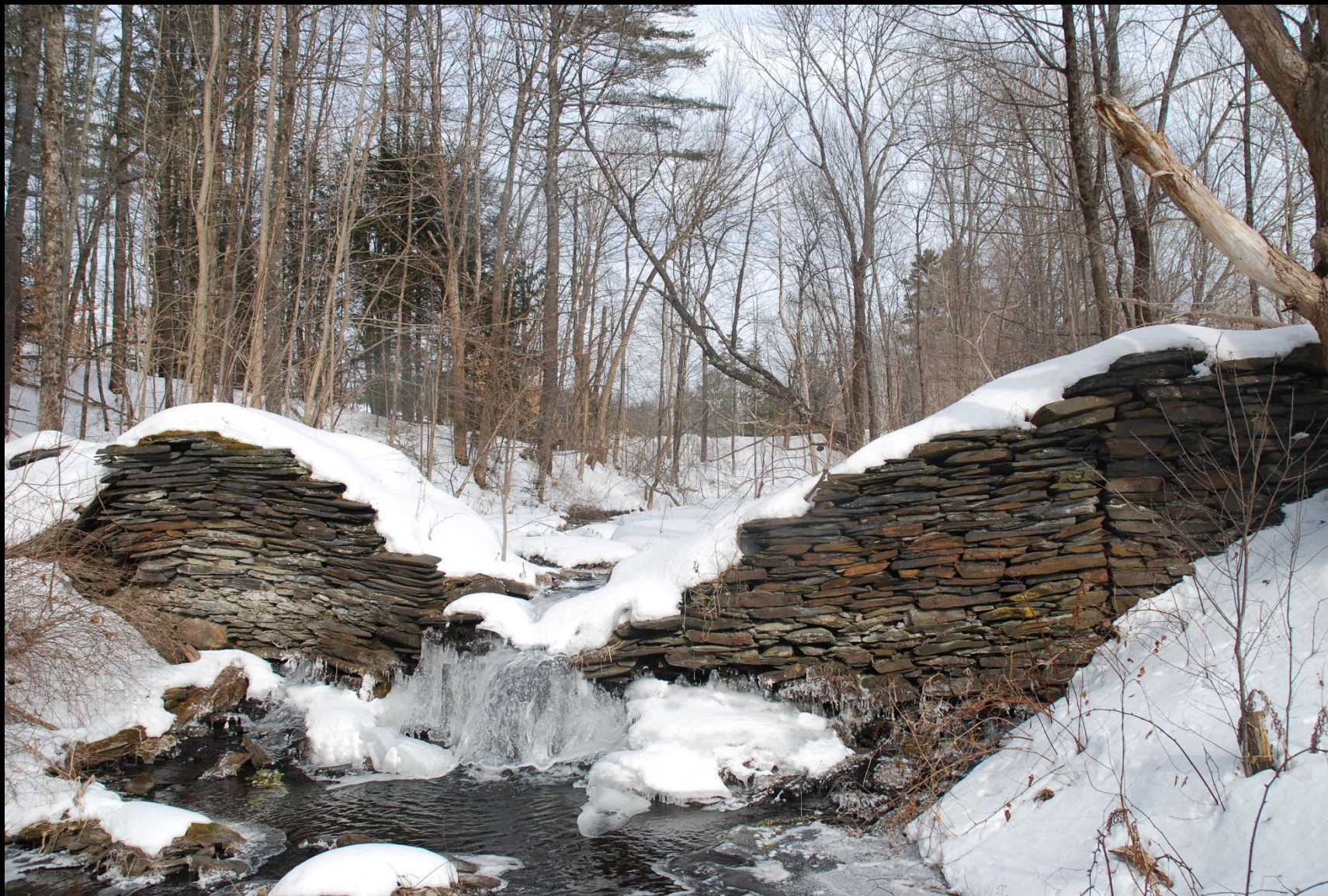
VT_Washington County_Maple Corner_026
