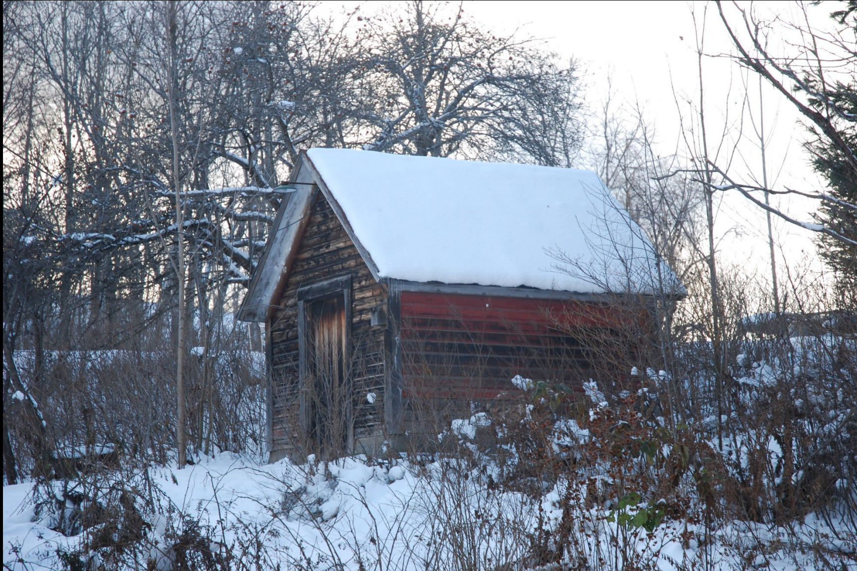
VT_Washington County_Maple Corner_021
