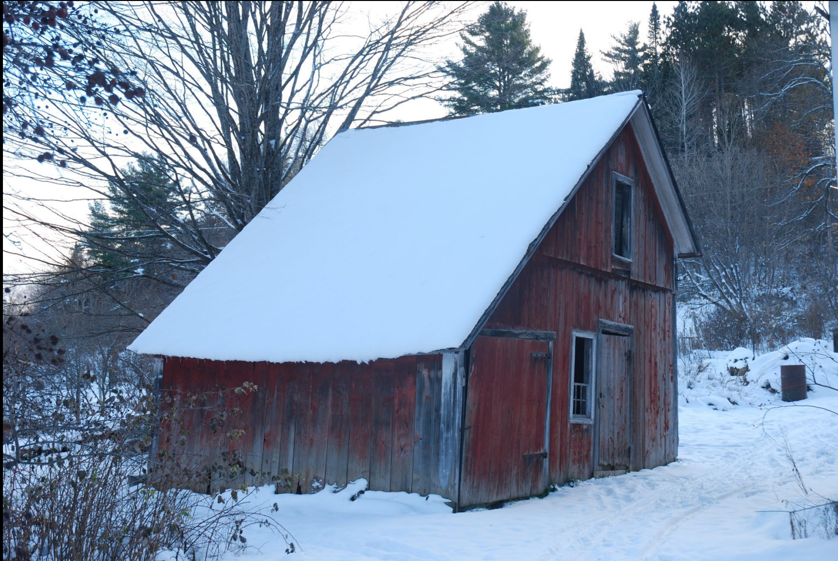
VT_Washington County_Maple Corner_020
