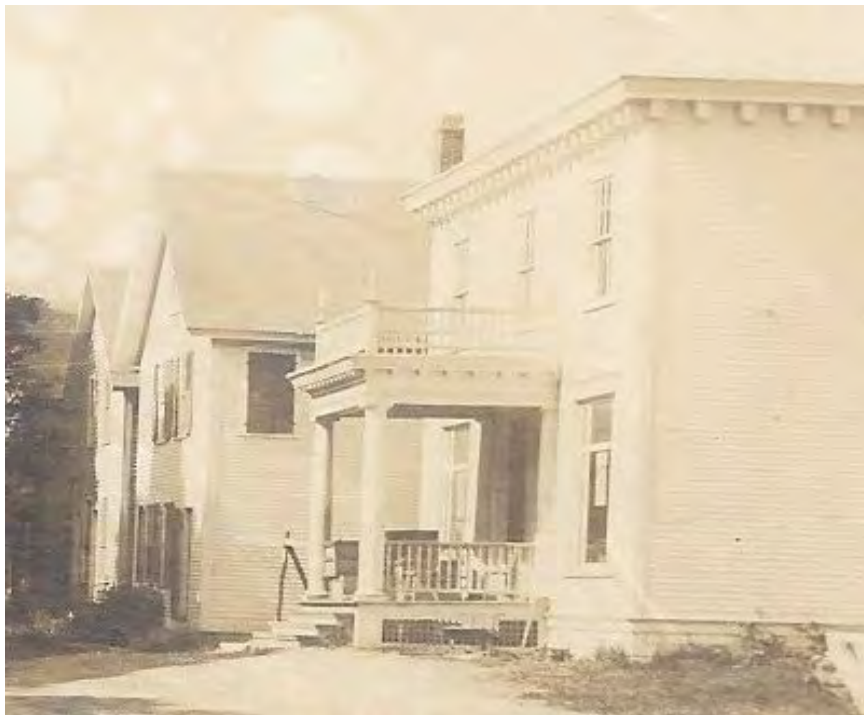
J.M. Griffith Store c1910. Main (aka Village) Street -formerly Bowen & Hopkins
