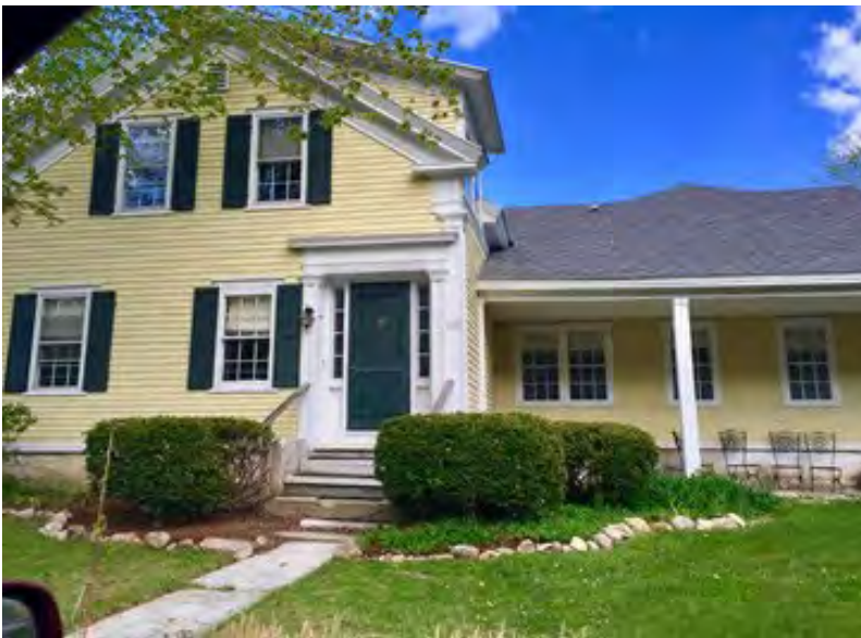
120 Village St, west façade & wing, 2021
