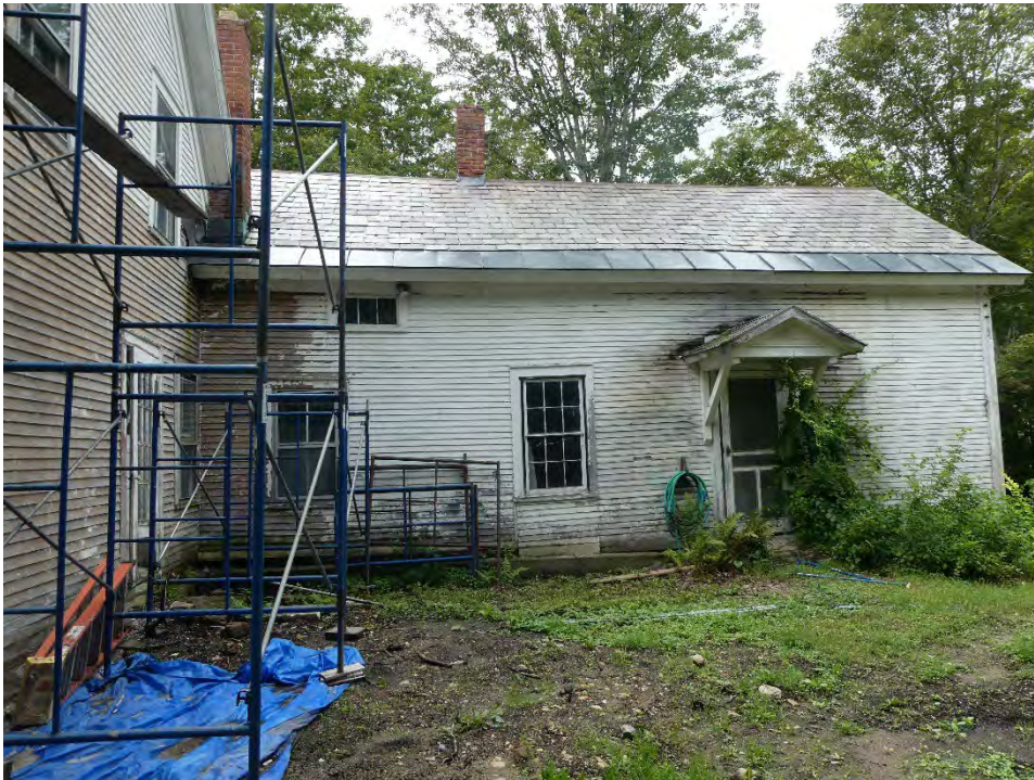
Rear of main block at left; extension north; looking west
