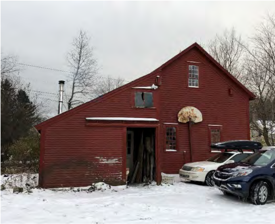
North façade of barn with saltbox profile, 2021
