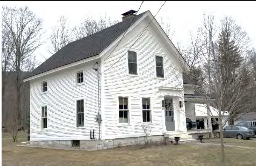
61 Pleasant St. View from the northwest, 2021, with contemporary garage to the rear and southeast. Michele Pagan
