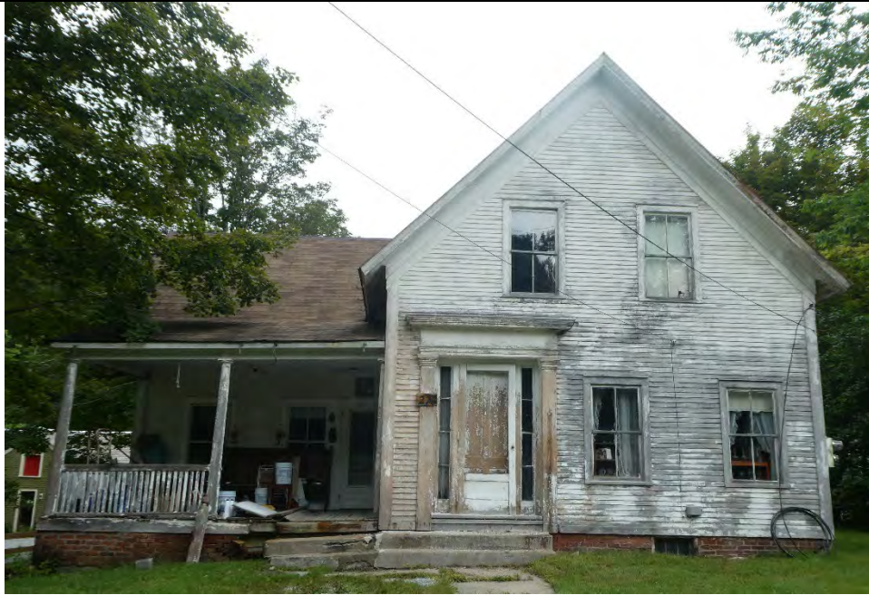
273 Mad Tom Road viewed from south - 2021
