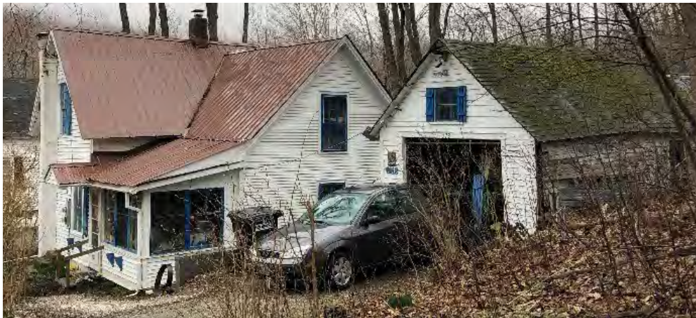
House viewed from southeast, with separate garage visible to the east.
