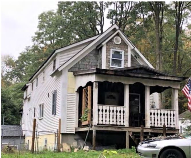
Façade from southwest corner. 2021
