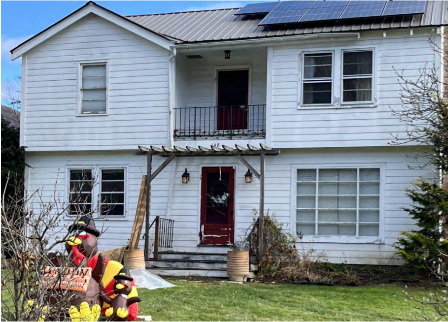
148 Village St. (2023). Solar panels added on roof.
