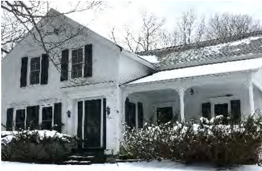
224 Mad Tom Rd, north-facing façade.
