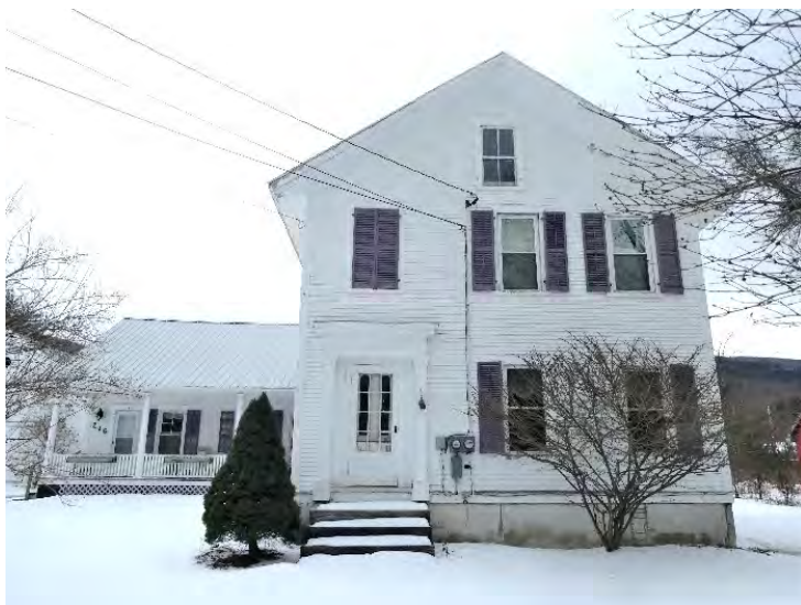
216 Village St., west façade and wing
