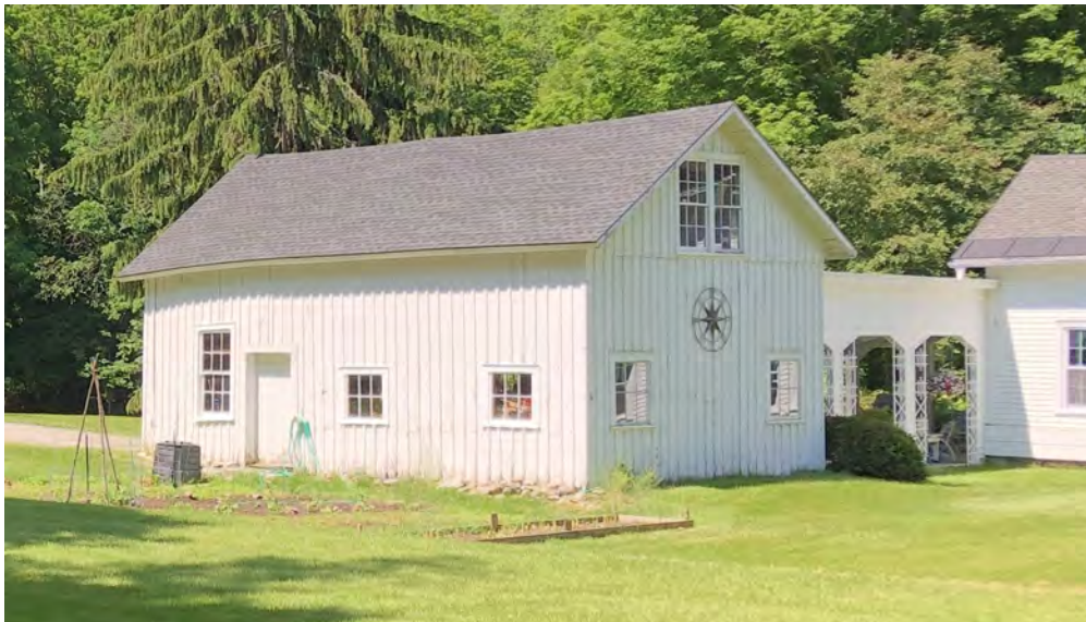
Ludlam garage, 2022, from Northeast.
