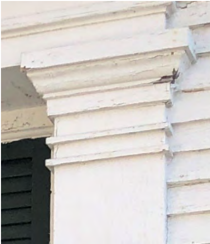
Ogee molding at top of column: later than the ¼-round molding seen on the 1852 Wilson House pilasters Michele.Pagan
