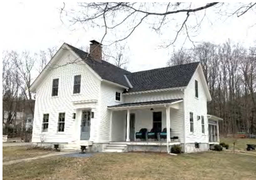
61 Pleasant St. west facade
