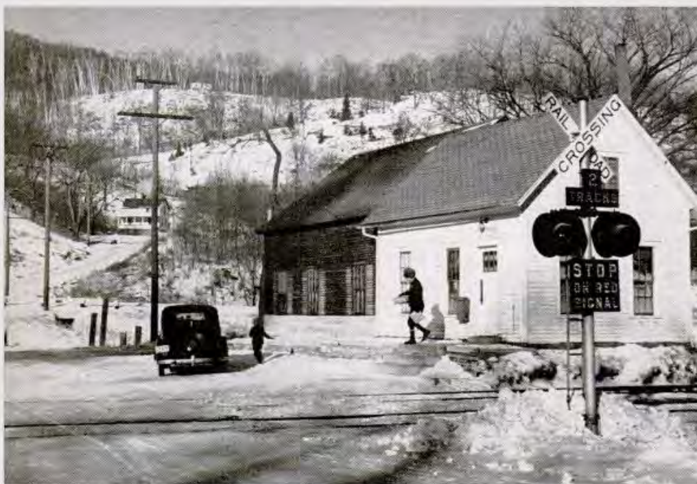
Mark Whalen leaves East Dorset post office ( above ) at 8:30 every morning but Sunday and drives 24 miles to visit 80 mailboxes. Rutland Railroad runs through the village.
