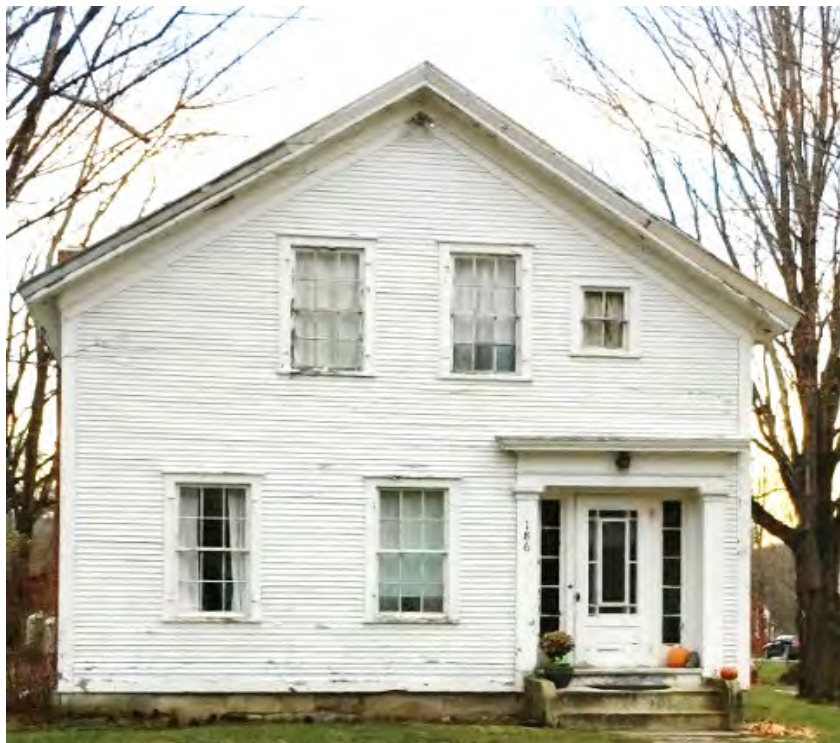
186 Mad Tom Road, north façade, 2021
