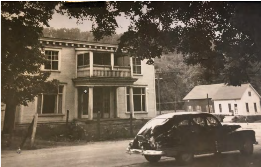
c1950 Enclosed double porch added
