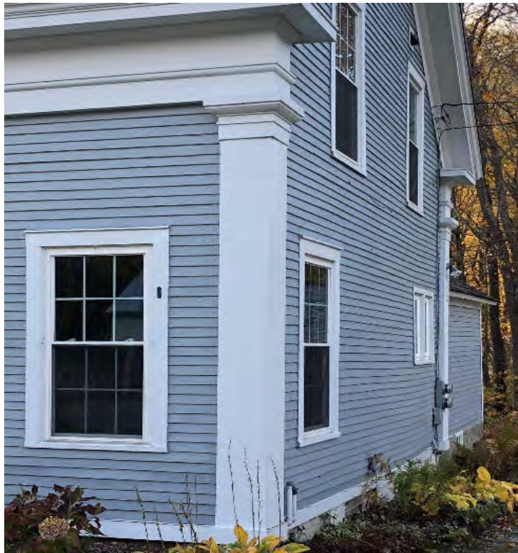
Northeast corner detail with quarter-round cap, 2021
