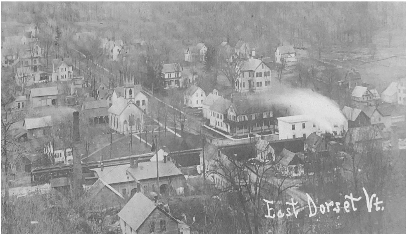
c1910 Village overview from the northwest. NOTE the white lines - (aka sidewalks) made from 'flat-backs,' end slabs first cut off blocks of quarried marble.
