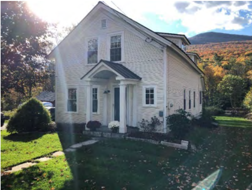
House from the northeast corner
