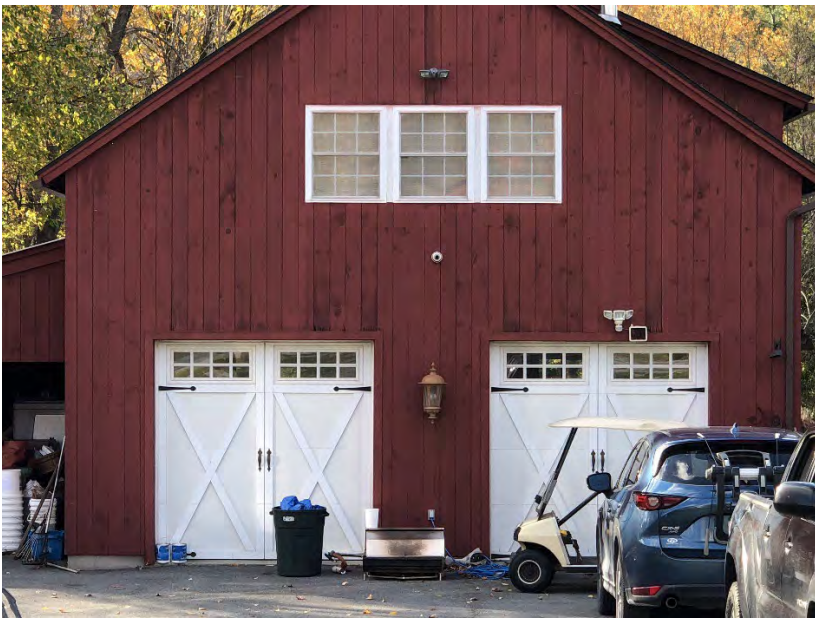
Two car garage with apartment above, east façade
