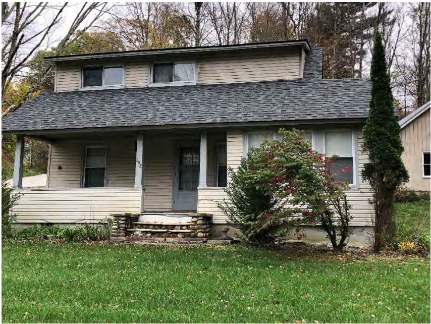
West facing façade - 2021
