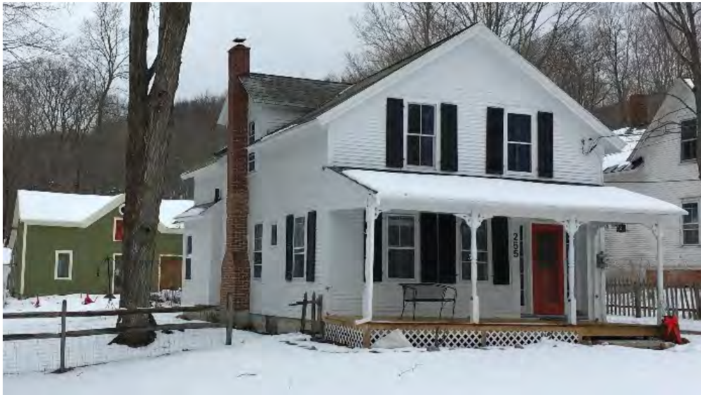
255 Mad Tom Road, south façade, 2021
