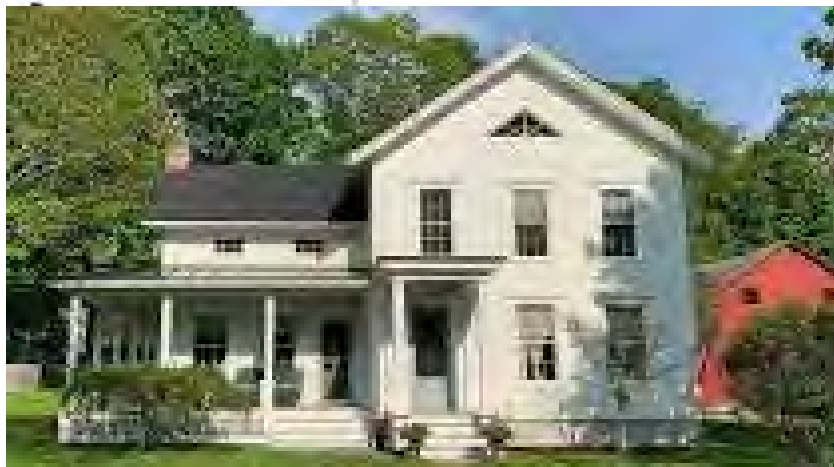
41 Pleasant St, west façade, with barn to southeast, 2021
