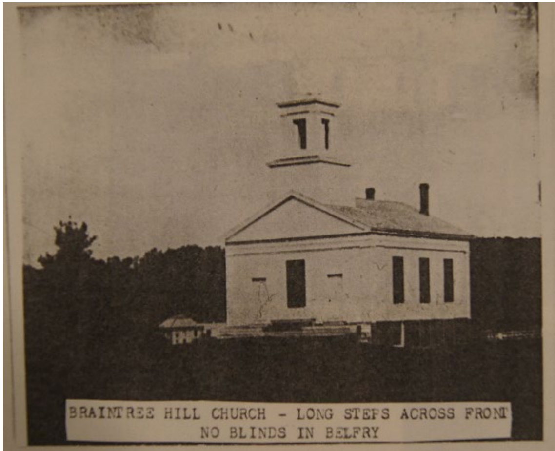
Figure 9: Undated photograph looking northwest toward Braintree Hill Meetinghouse. Note long granite steps across front, no blinds in belfry. On east basemen wall it appears that a stove pipe may be extending from basement ventilation arch. Collections of the Braintree Historical Society.
