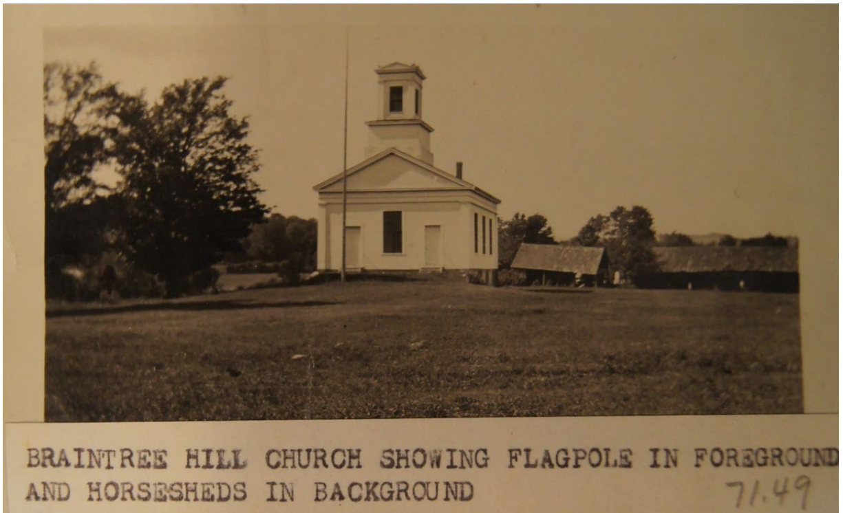
Figure 10: Undated photograph (pre-1930s) looking north to Braintree Hill Meetinghouse. Collections of the Braintree Historical Society.
