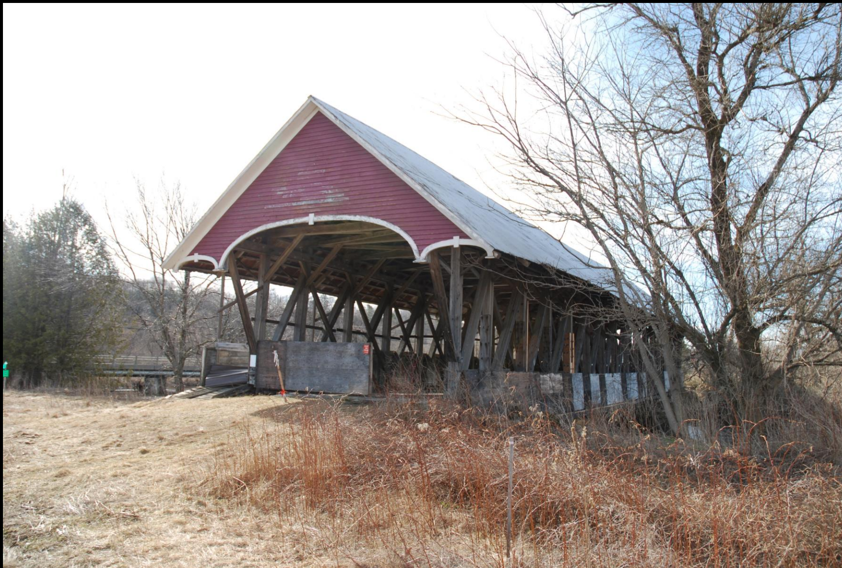
VT_Caledonia County_Centre Covered Bridge_004
