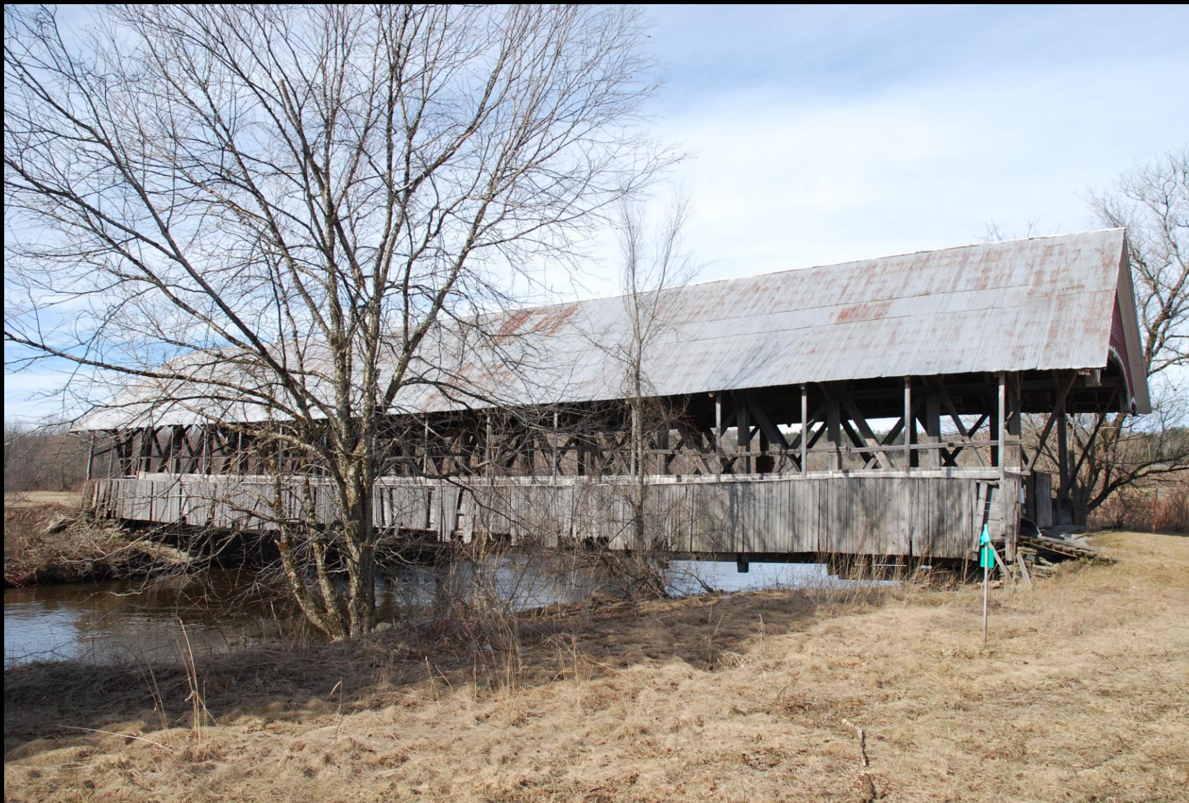
VT_Caledonia County_Centre Covered Bridge_006
