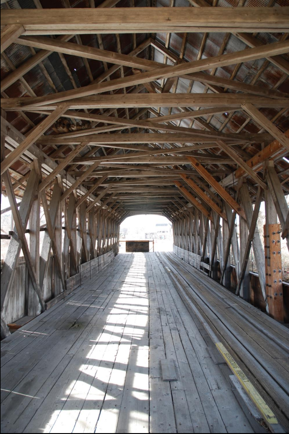
VT_Caledonia County_Centre Covered Bridge_010
