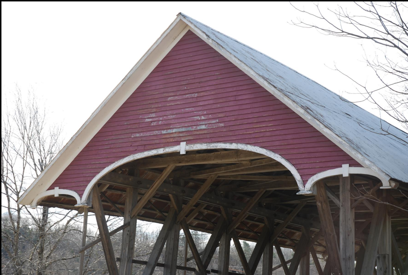
VT_Caledonia County_Centre Covered Bridge_005
