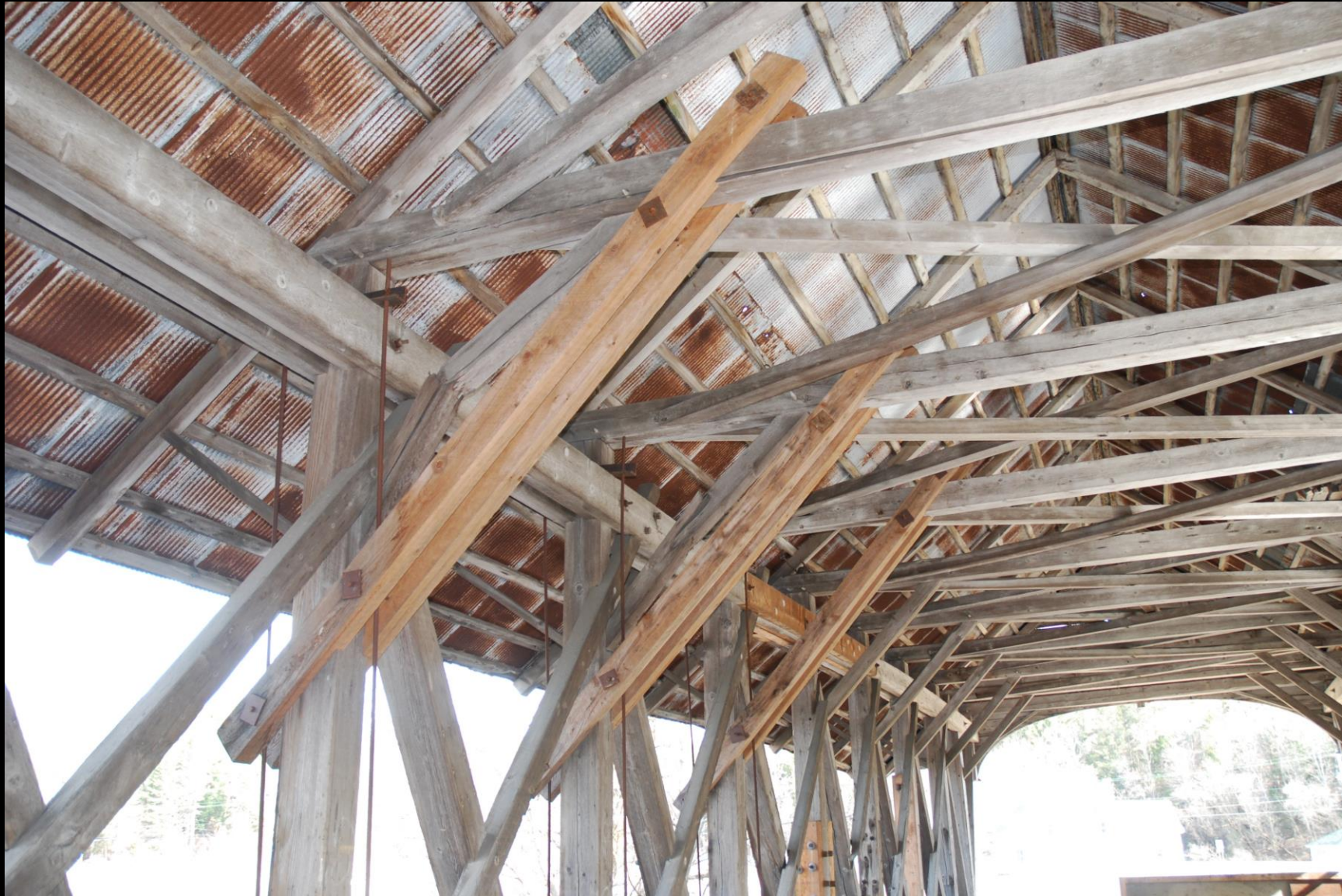
VT_Caledonia County_Centre Covered Bridge_013
