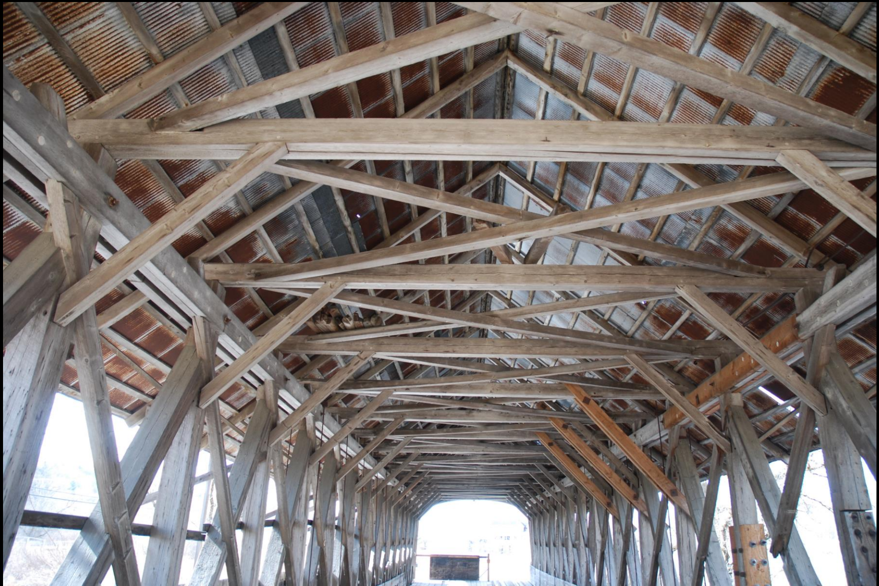
VT_Caledonia County_Centre Covered Bridge_009
