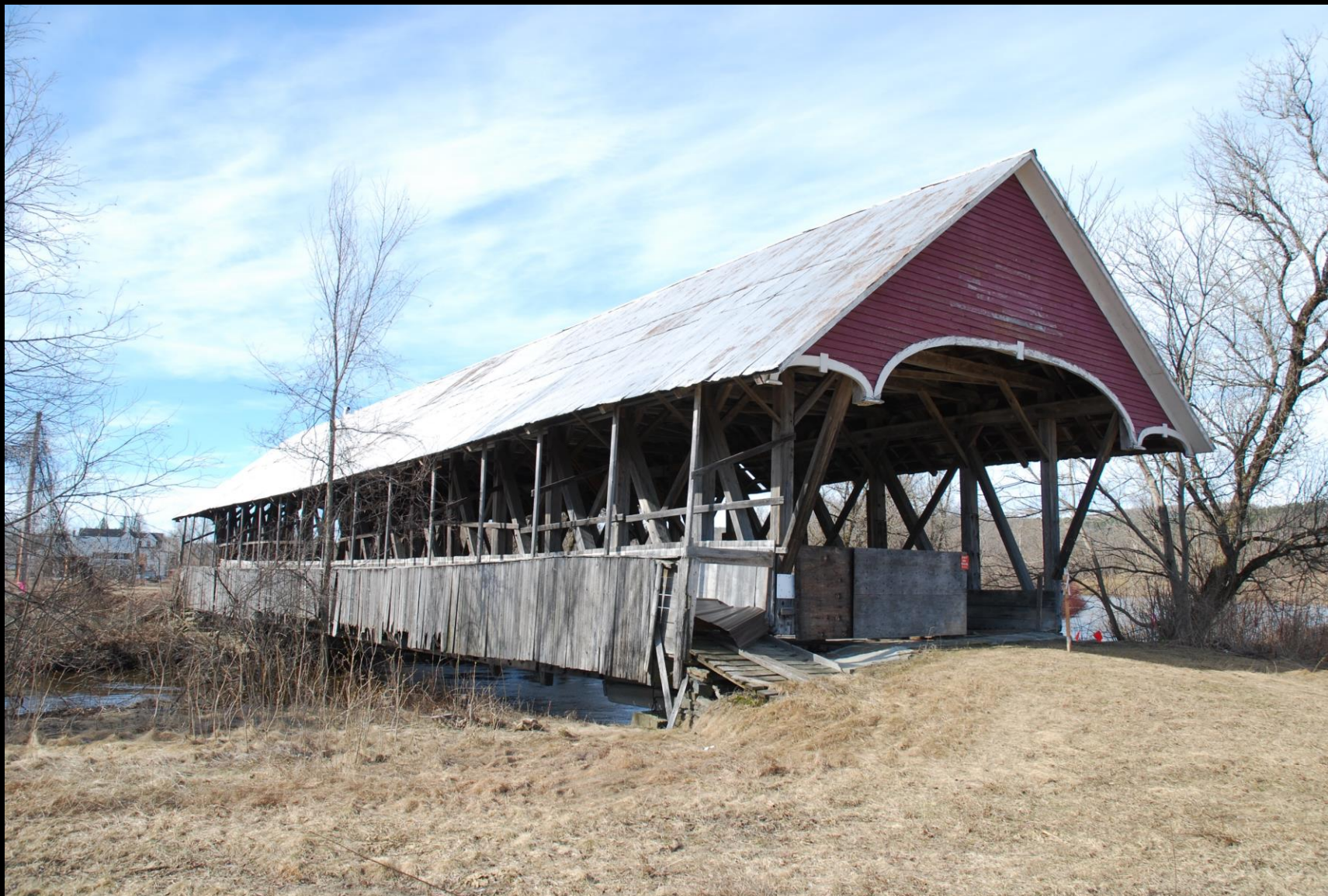
VT_Caledonia County_Centre Covered Bridge_003
