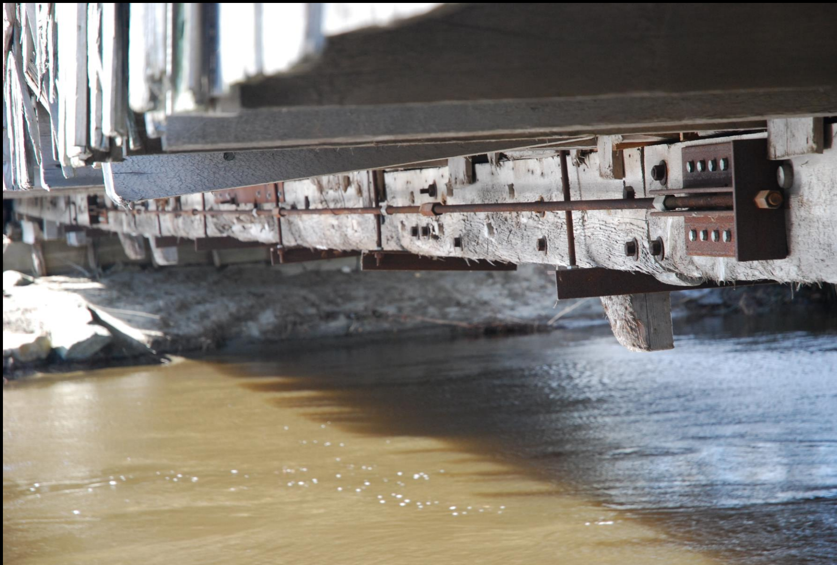
VT_Caledonia County_Centre Covered Bridge_008
