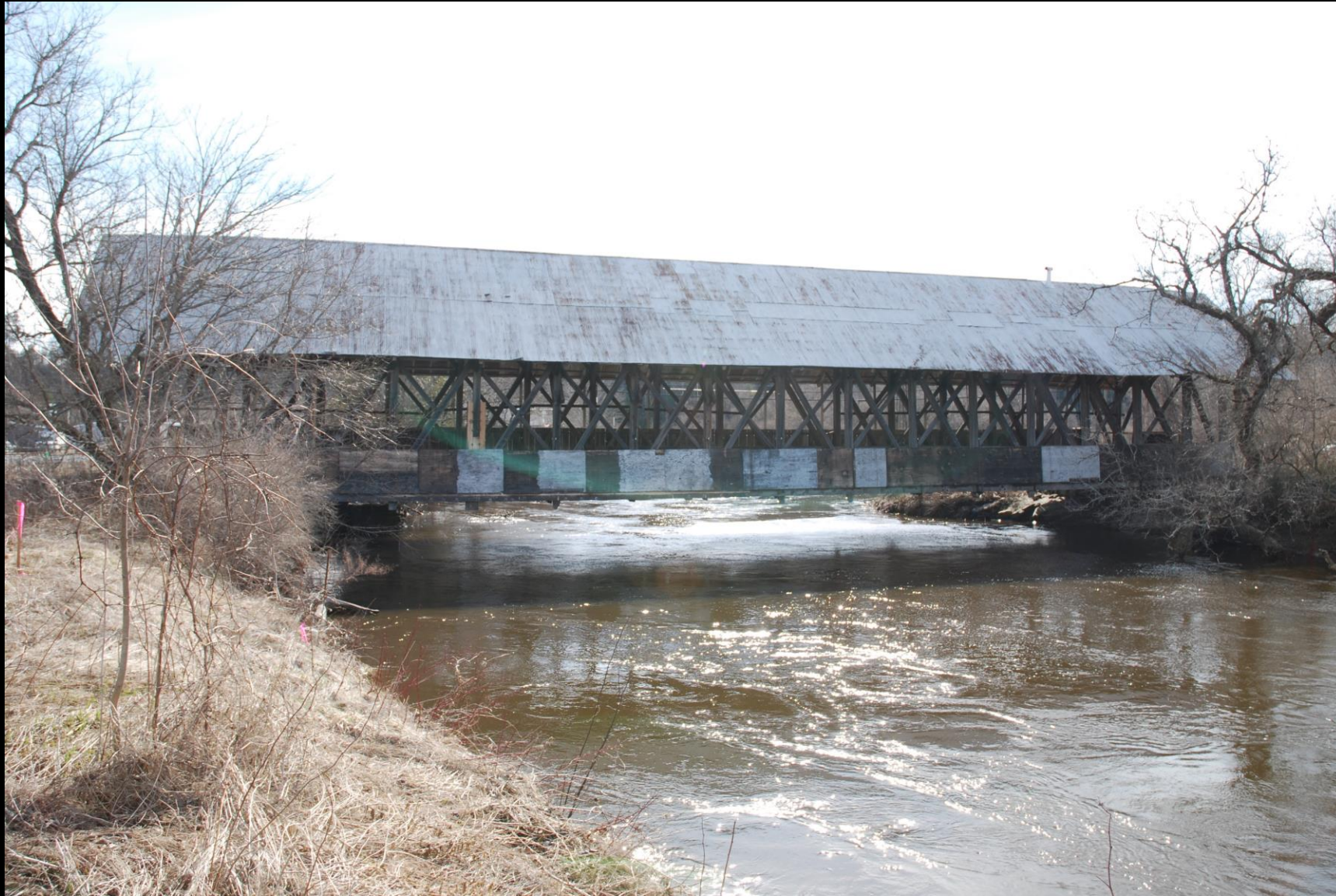
VT_Caledonia County_Centre Covered Bridge_007
