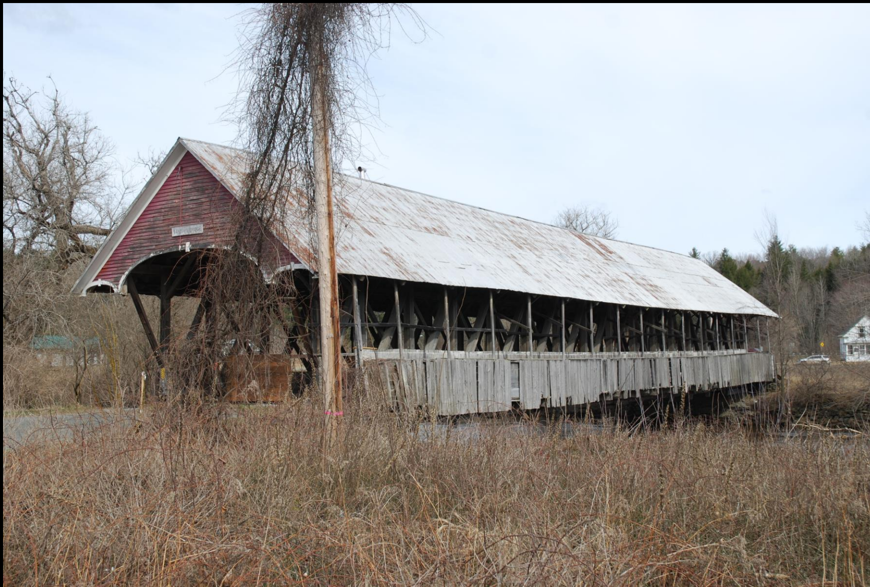
VT_Caledonia County_Centre Covered Bridge_001
