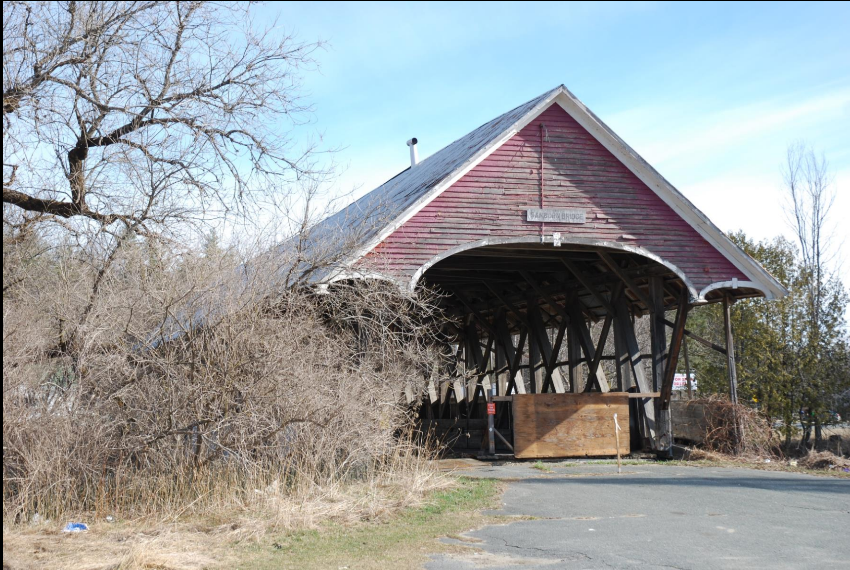
VT_Caledonia County_Centre Covered Bridge_002
