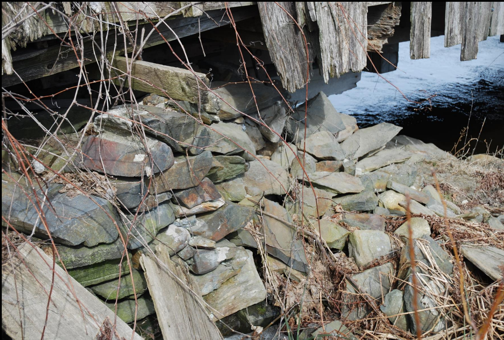
VT_Caledonia County_Centre Covered Bridge_015
