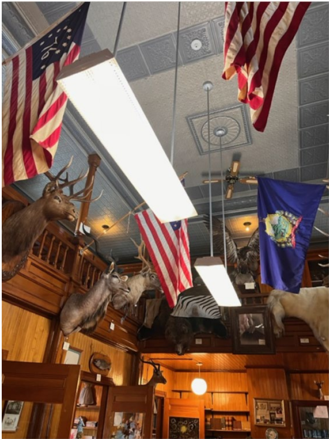
2023 – pressed metal ceiling
