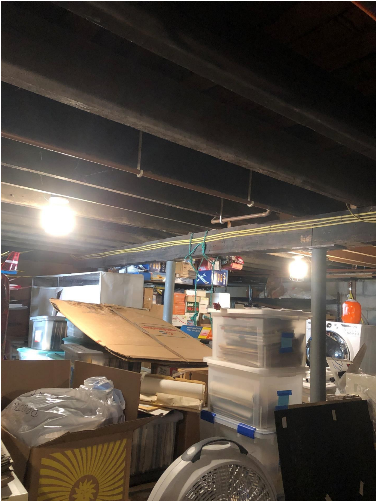
Basement framing in house. Sawn dimensional lumber with a built-up center beam.
