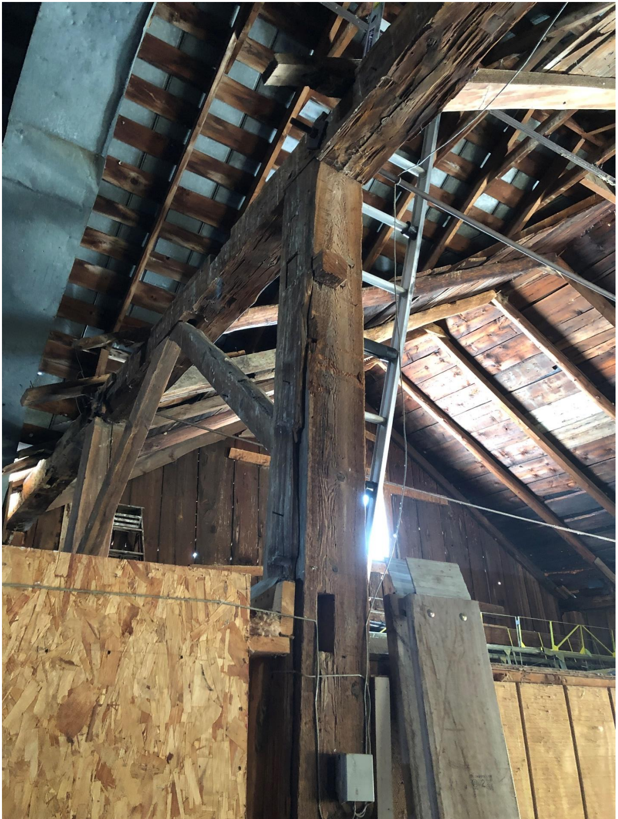
Detail of timber framing in east barn
