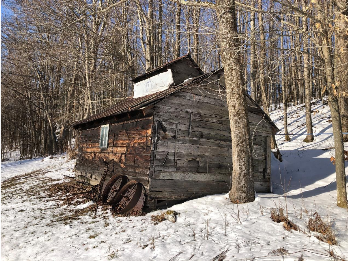
View looking southwest at sugarhouse, with sugarbush
