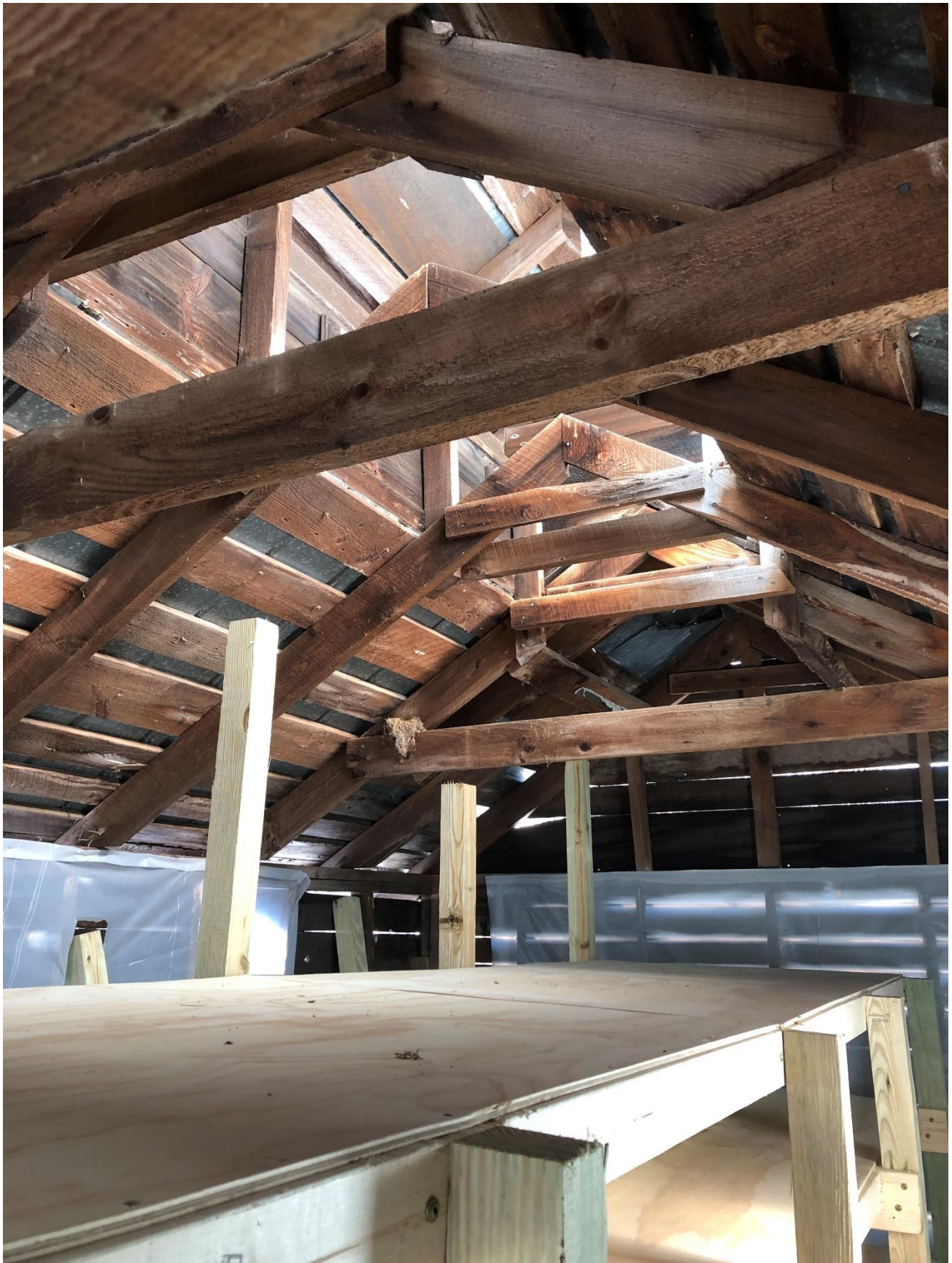
Interior view of sugarhouse and roof monitor
