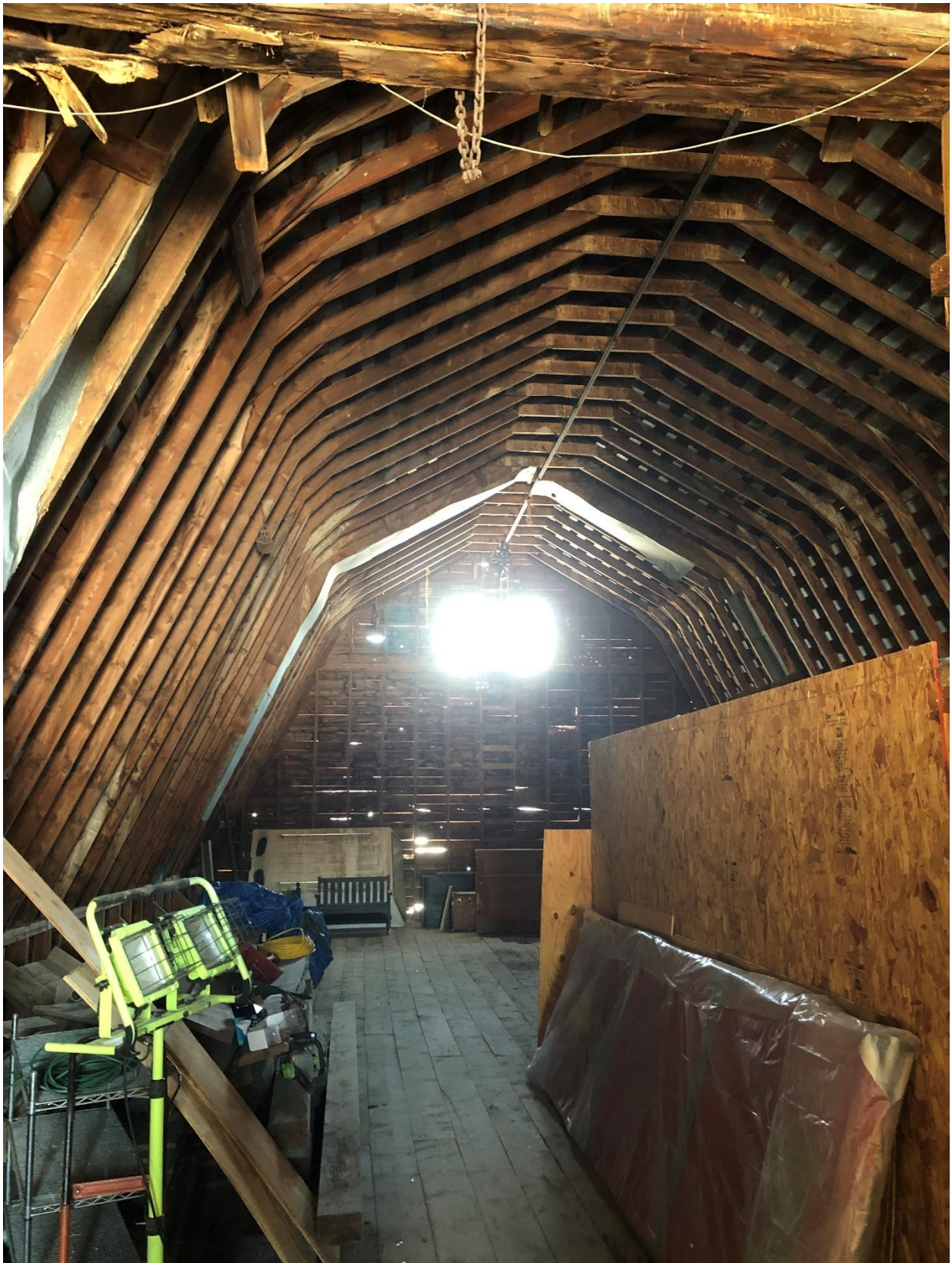
Hayloft in gambrel roof barn addition
