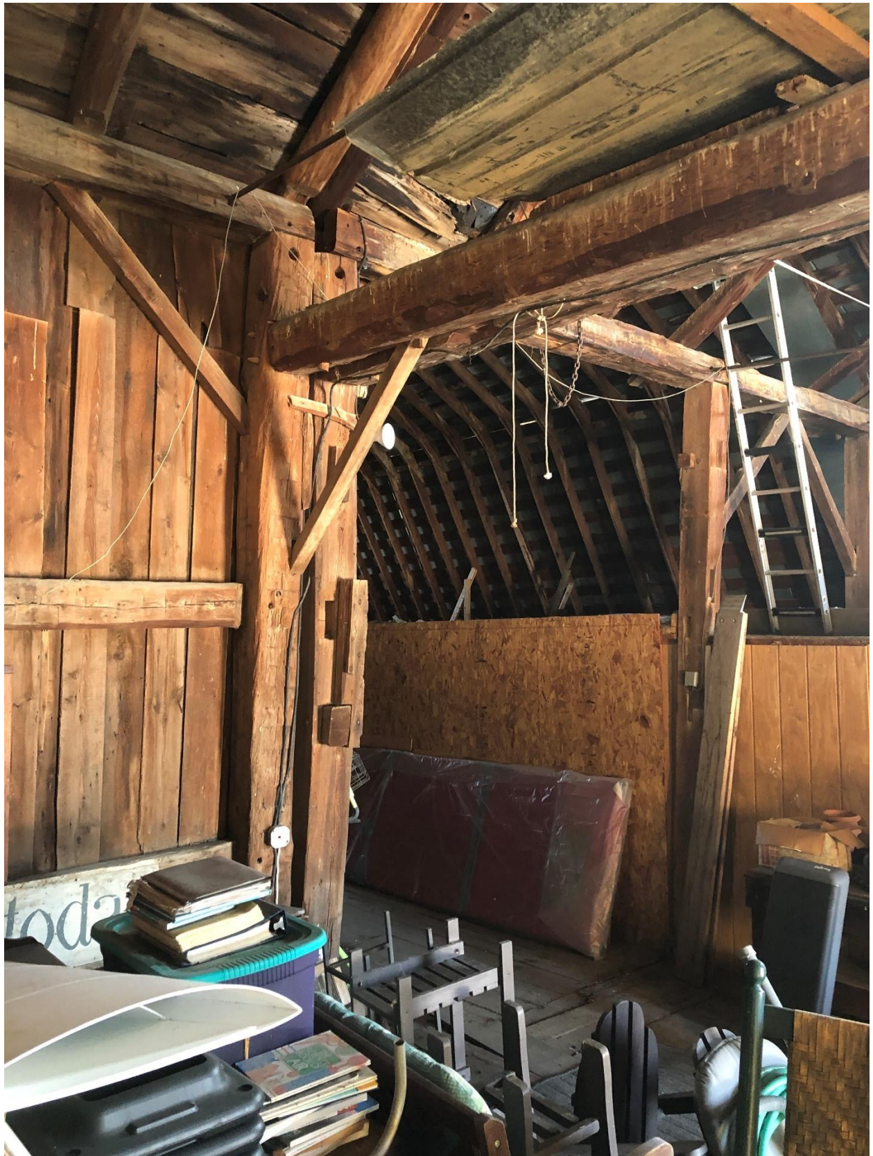
Barn framing an junction of east and west barns (note double corner posts) with gambrel roof barn in the background.
