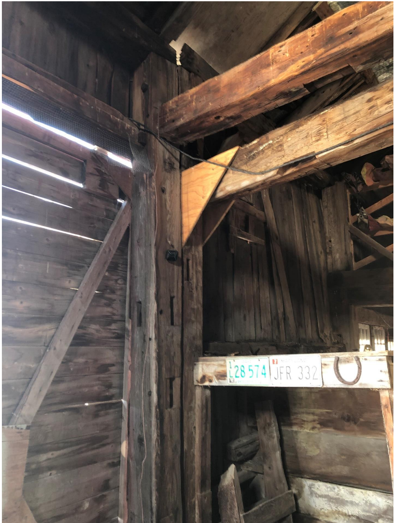
Detail of timber frames in east and west barns
