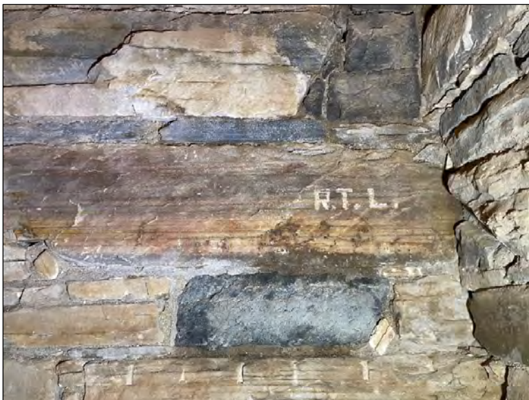
Figure 3. Typical interior coursed rubble masonry. Note color difference between stones.
