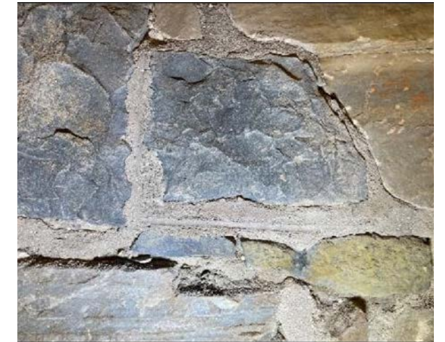
Image 30. Typical interior condition. Jablonski
