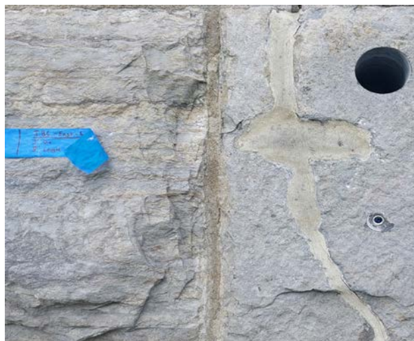
Image 74. Caulk repair and current core hole
