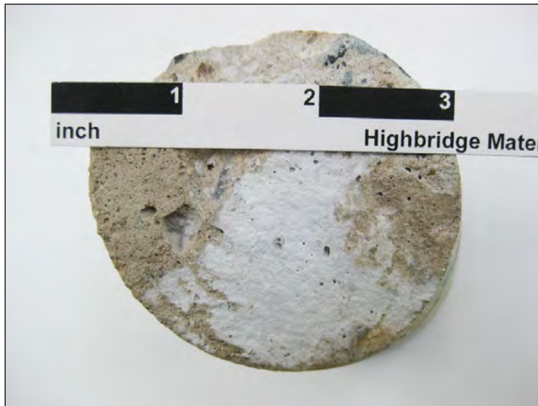
Figure 35. Formed end of core sample ANA-South-4 showing a thin white residue consisting of alkali-aggregate reaction gel.
