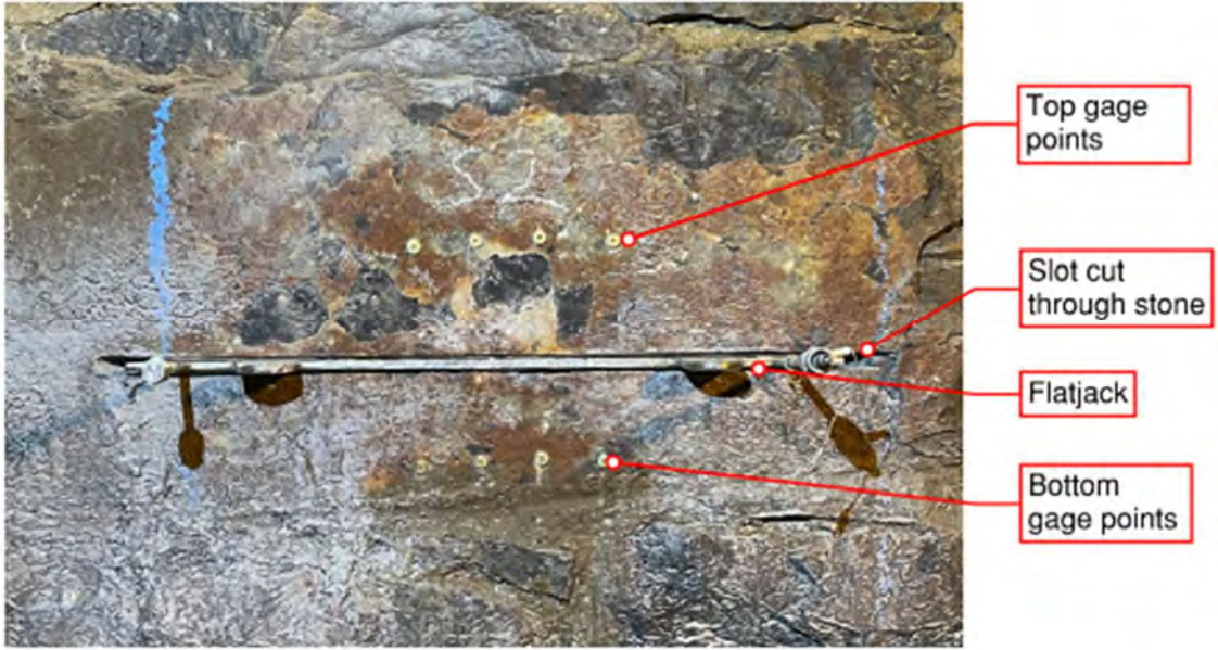
Figure 31. Typical Stress Test Setup
