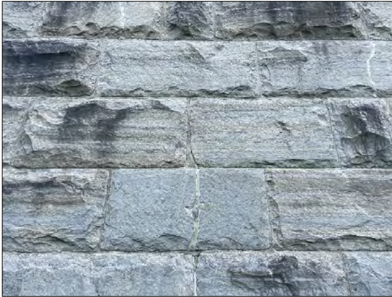
Figure 2. Typical exterior rock-faced, coursed Sandy Hill dolomitic limestone ashlar.
