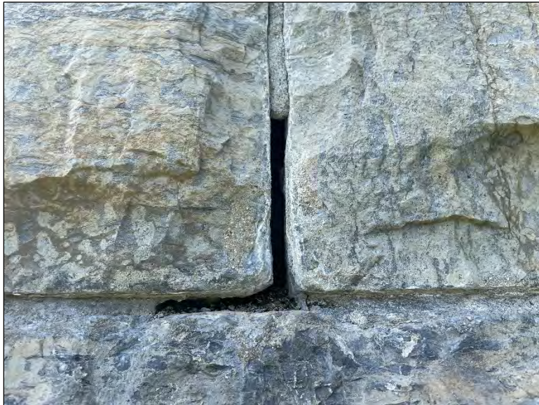
Figure 32. Sampling location for BM-01 (open joint).
