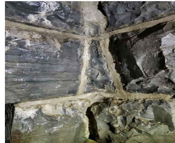
Image 87. Corner condition at top of monument. Stevens & Associates
