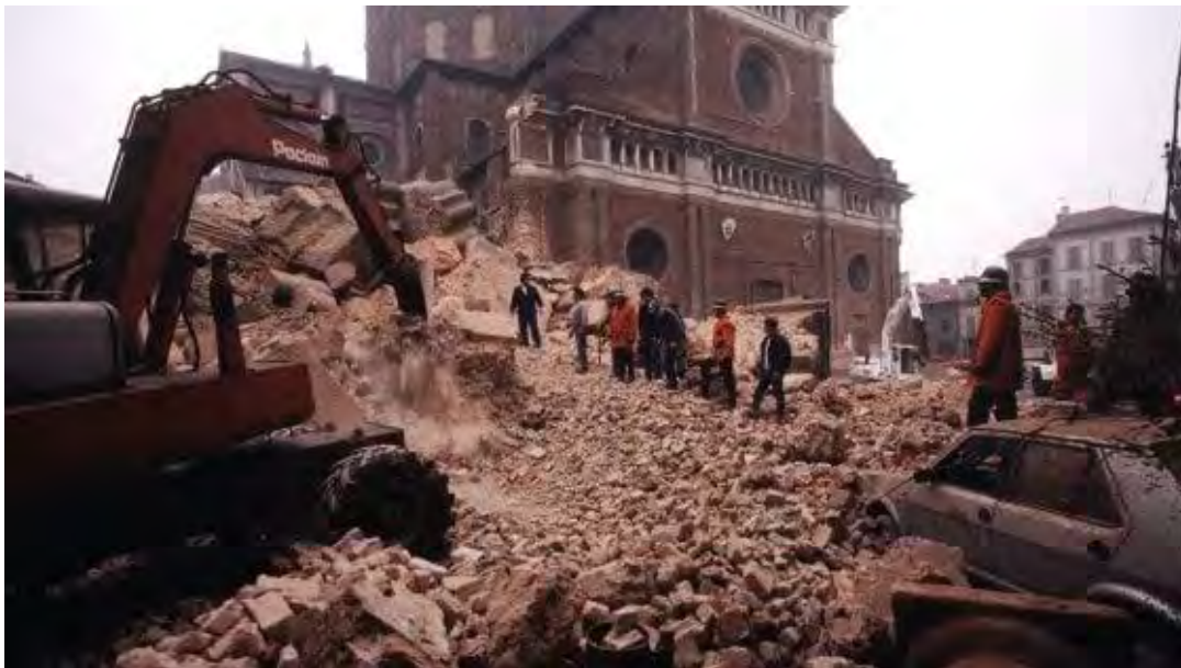
Figure 1 Pavia Tower Collapse [2]
