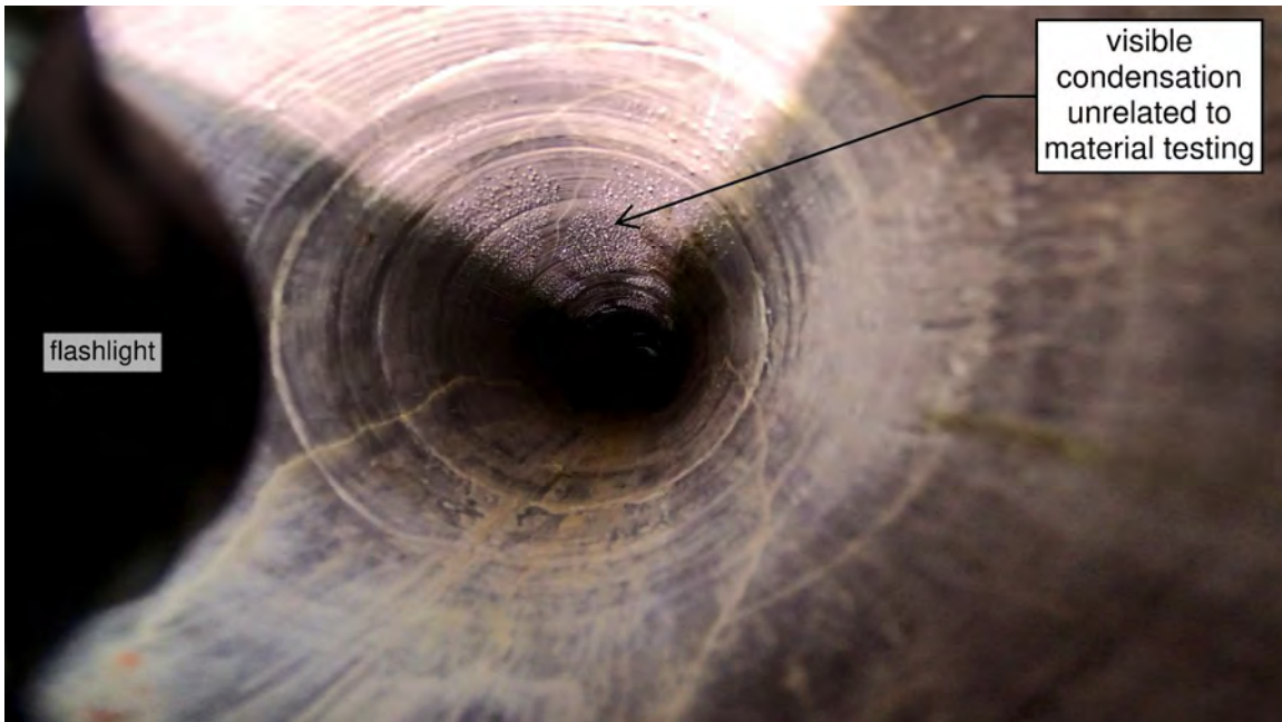
Figure 18. GoPro photo of the internal wythe at CORE-SOUTH after the Goodman Jack testing. The stone is visibly intact. There is visible condensation at the top of the core hole for much of the depth of CORE-SOUTH unrelated to the material testing.
