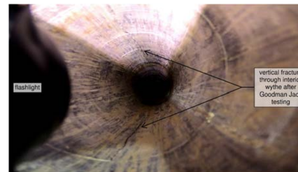
Image 18. Interior face wythe, CORE-NORTH after Goodman Jack testing. Atkinson-Noland & Associates
