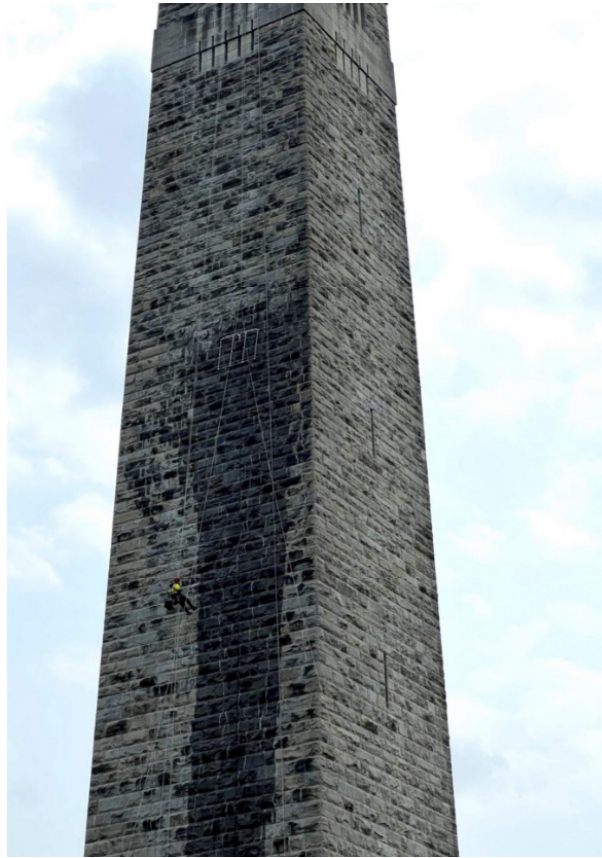
Image 26. North Elevation. Atkinson-Noland & Associates
