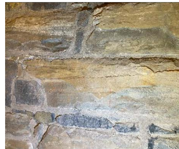
Image 32. Typical interior condition. Jablonski
