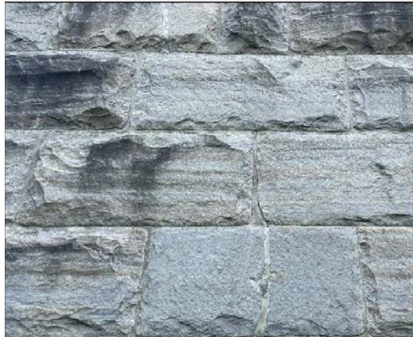
Image 72. Typical exterior rock-faced, coursed Sandy Hill dolomitic limestone ashlar. Jablonski
