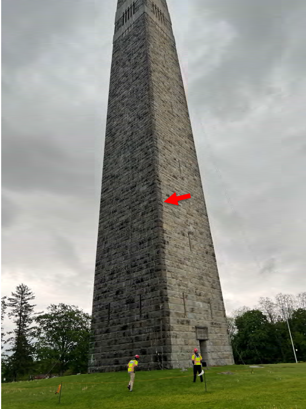
Figure 27. Photo of north wall following rainstorm with the prevailing wind coming directly from the north. The monument largely blocked wind driven rain from the leeward walls, with a small amount of moisture being blown and wrapping around the corners of the monument creating a clear line of moisture approximately half the length of a stone unit to the east and west elevations.
