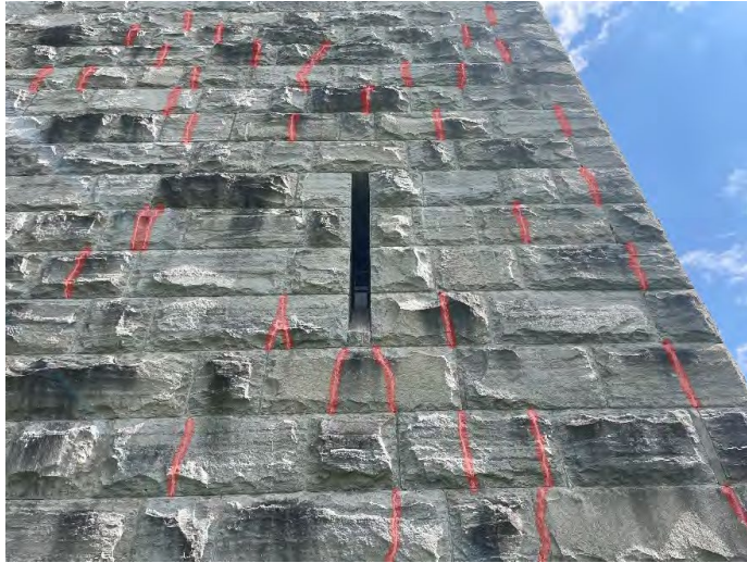
Exterior Cracks in Red (over 6,300 noted)
