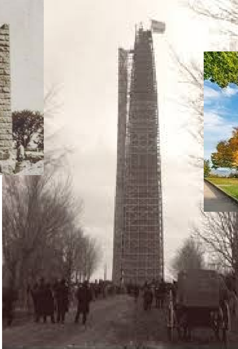
In progress construction images of monument
