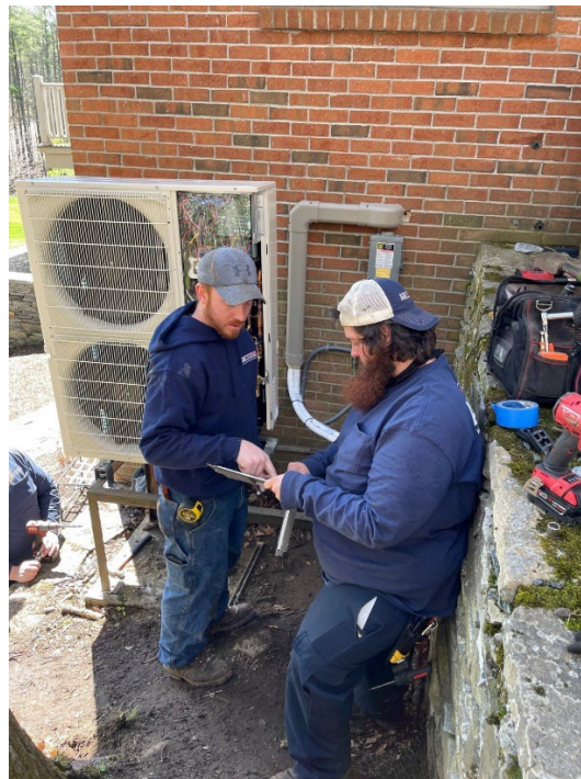
Image Caption: Employees working on an HVAC system.
