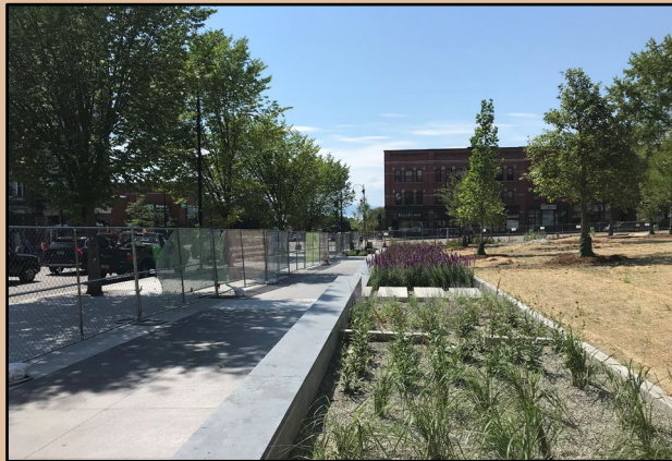
Stormwater improvements on Main Street which were constructed as part of the contract for City Hall Park.
