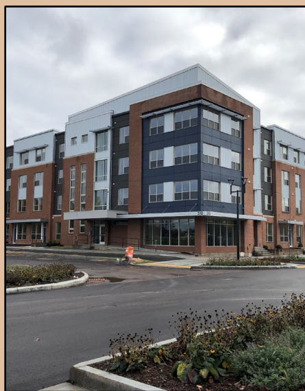
Garden Street apartments nearing construction completion in the Fall of 2019, with completed Market and Garden Street improvements.
