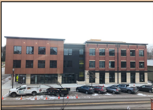
Completed redevelopment of Core Brownfield Site #3 – Congress and Main Streets. Photo provided St. Albans City.
