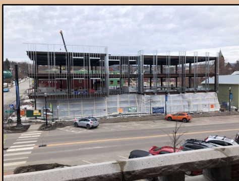
Remediation and redevelopment in progress at Core Brownfield Site #3 – Congress and Main Streets. Photo provided by Chip Sawyer, St. Albans City.
