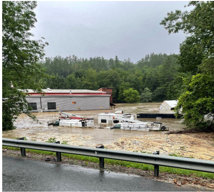
Floodwater inundates a warehouse and service vehicles
