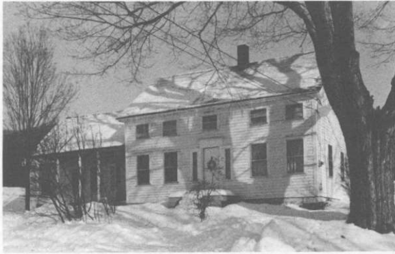
This house (2), located in the northwest corner of Mendon, was one of a number of farmhouses built in the western portion of town in the years before 1860. Dating from c.1830, it is a good example of an early Classic Cottage. Noteworthy details include the kneewall windows, marble block foundation, and a central doorway with sidelights and a simple Federal style entablature.
