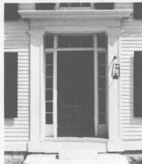
Constructed c.1845, this house (5) is a typical Classic Cottage in form, but it is unusual in that the walls are built of stacked planks of wood. The central door is framed by a Greek Revival style surround with a transom, full-length sidelights, and paneled pilasters which match those on the corners of the house.
