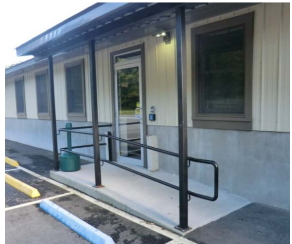
Figure 10: Dead River Propane offices have sealed walls and door dams to keep floodwaters out
