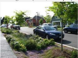
ABOVE: A shallow bio-swale with a variety of plants is used in place of lawn in a tree-island next to a road to achieve an attractive border that reduces flooding and improves water quality.
