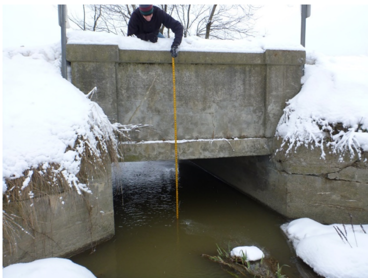
Figure 4.3: Fieldwork Makes the Difference – Measuring Undersized Culvert
