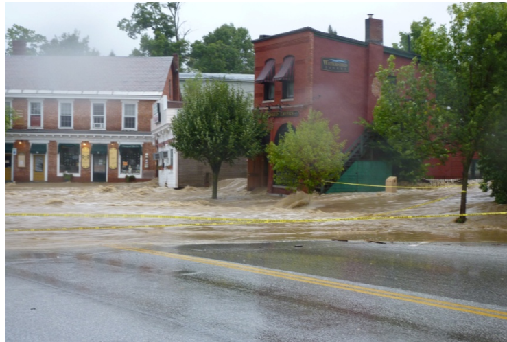
Figure 5: Flooding in downtown Brandon during Tropical Storm Irene (Janet Mondlak, 2011)
