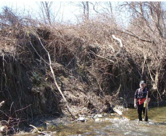
Mass failure before restoration
