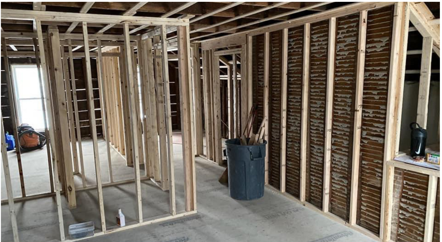
Exposed studs during a gut rehab and conversion of a historic home by small scale developer Zak Hale of Hale Resources in Bennington, Vermont. Photo Credit: Zak Hale.
