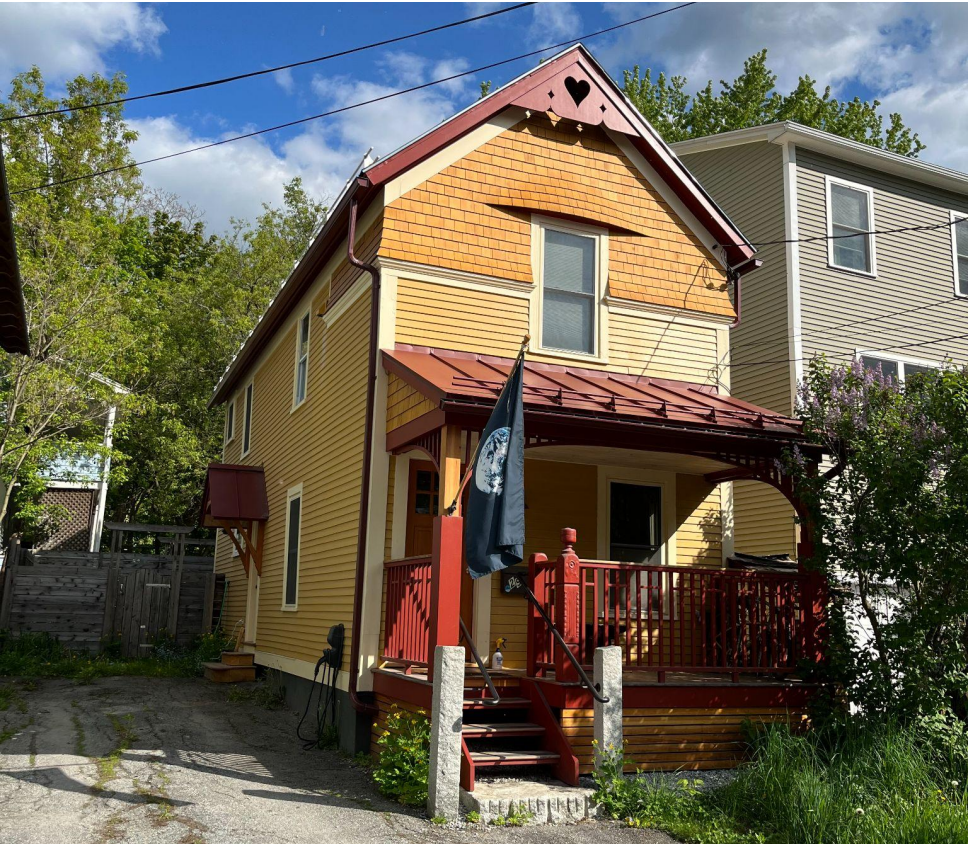
Franklin Street - Montpelier
