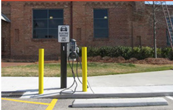
Figure 3. Over-protection can hinder accessibility of charging stations
