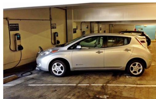
snow removal needs. In addition, many garages have power available and wall or ceiling mounting options which reduce installation cost. Fees for EV charging can be included in parking costs – some manufacturers offer charging equipment payment systems which can integrate with garage tickets. Other installation considerations as detailed in the perpendicular parking section will generally apply.
