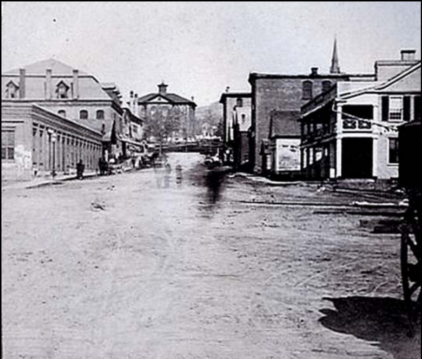
Lake Street Looking East
