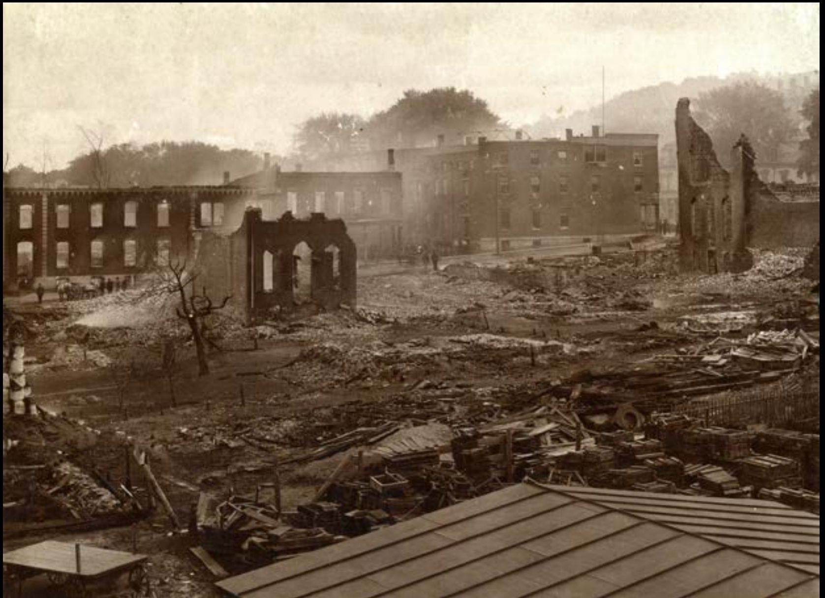
Looking Northeast From The Foundry
