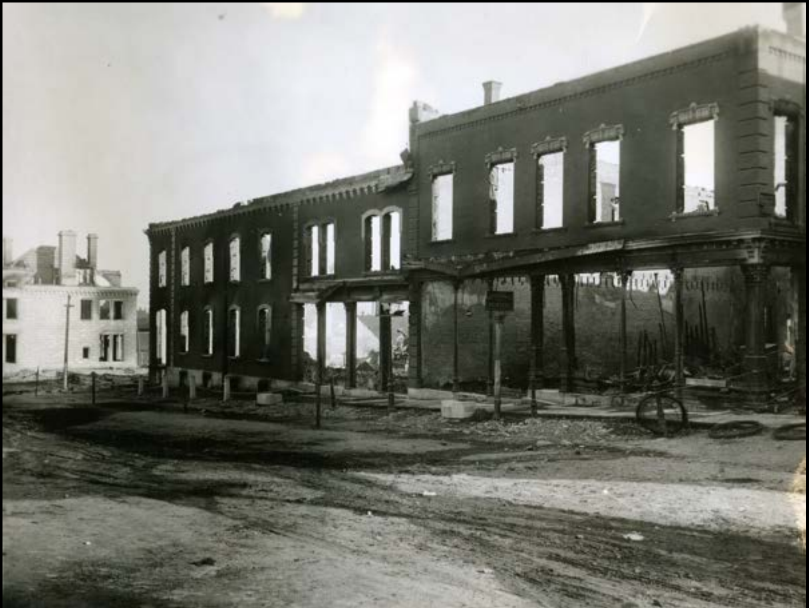
Kingman Street Looking At Messenger Building
