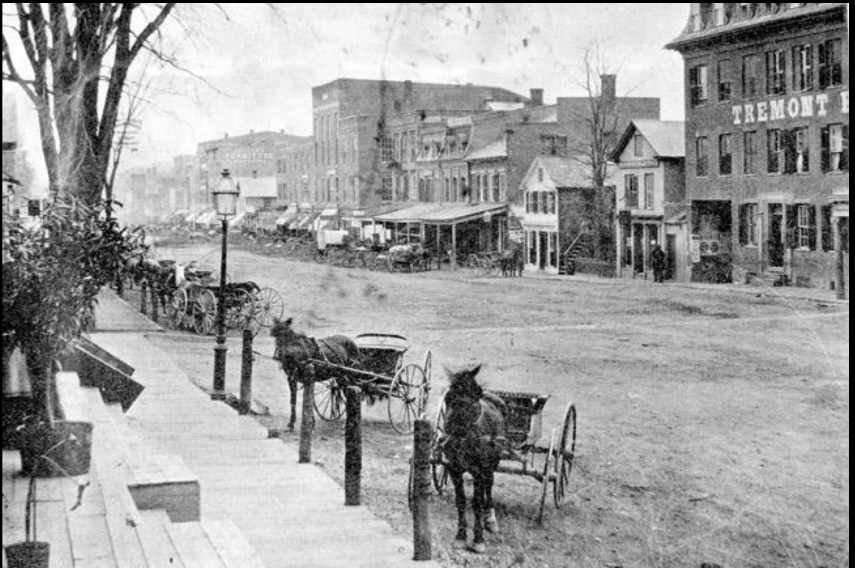
Corner of Main and Congress Street Looking South
