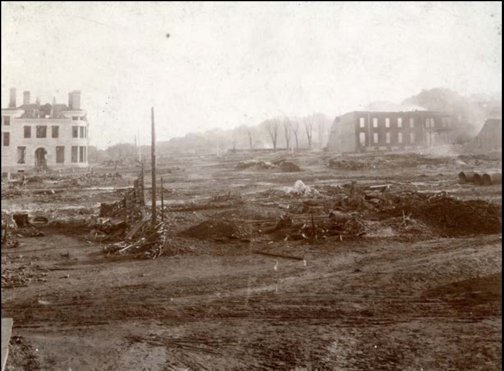
Looking North At Kingman Street
