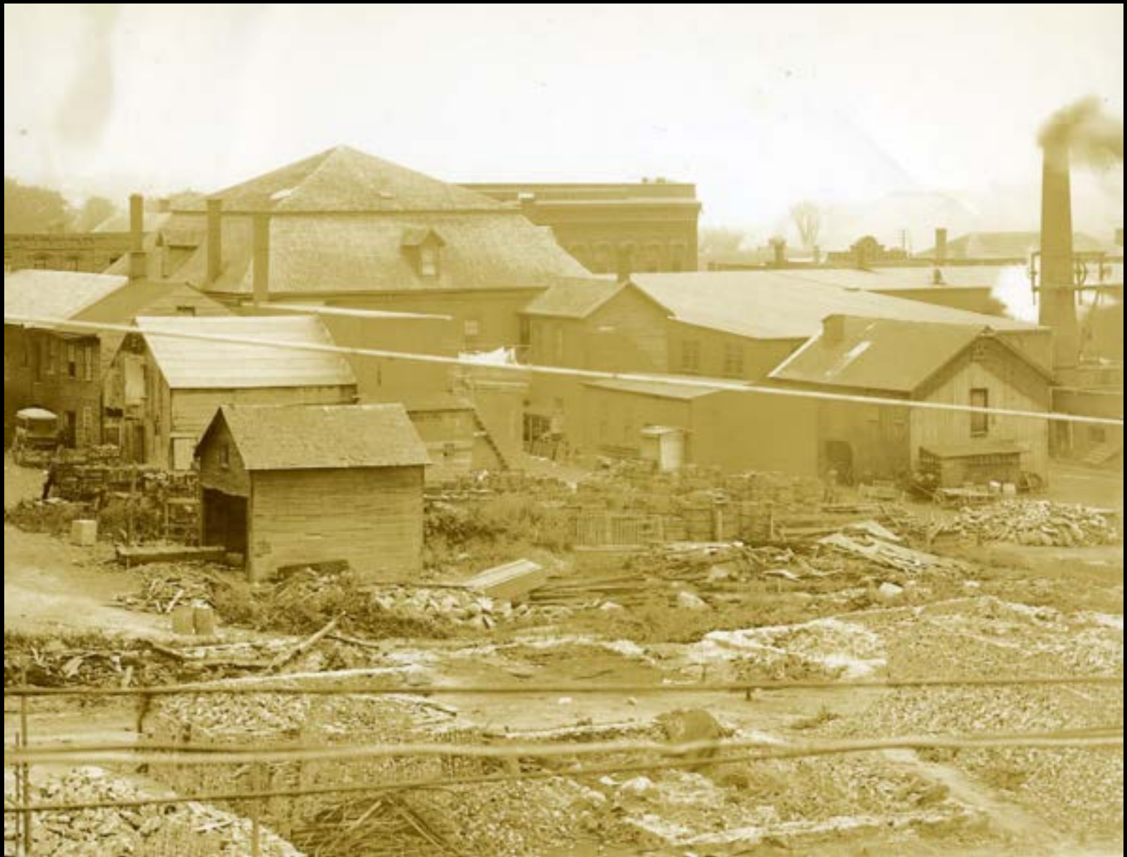
Looking South From Kingman Street
