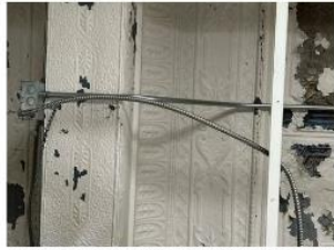
PHOTO OF EXISTING BEAM WRAP & BORDER
