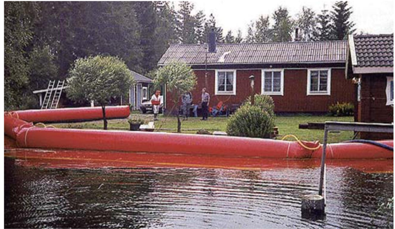
Inflated flood tubes as temporary barriers
