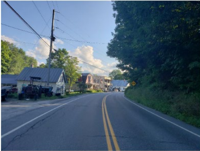
A: Eastern Approach to Village (VT Route 25)
