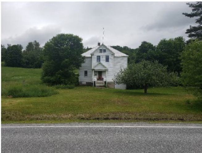
F: Waits River Schoolhouse, listed on the the National Register of Historic Places
