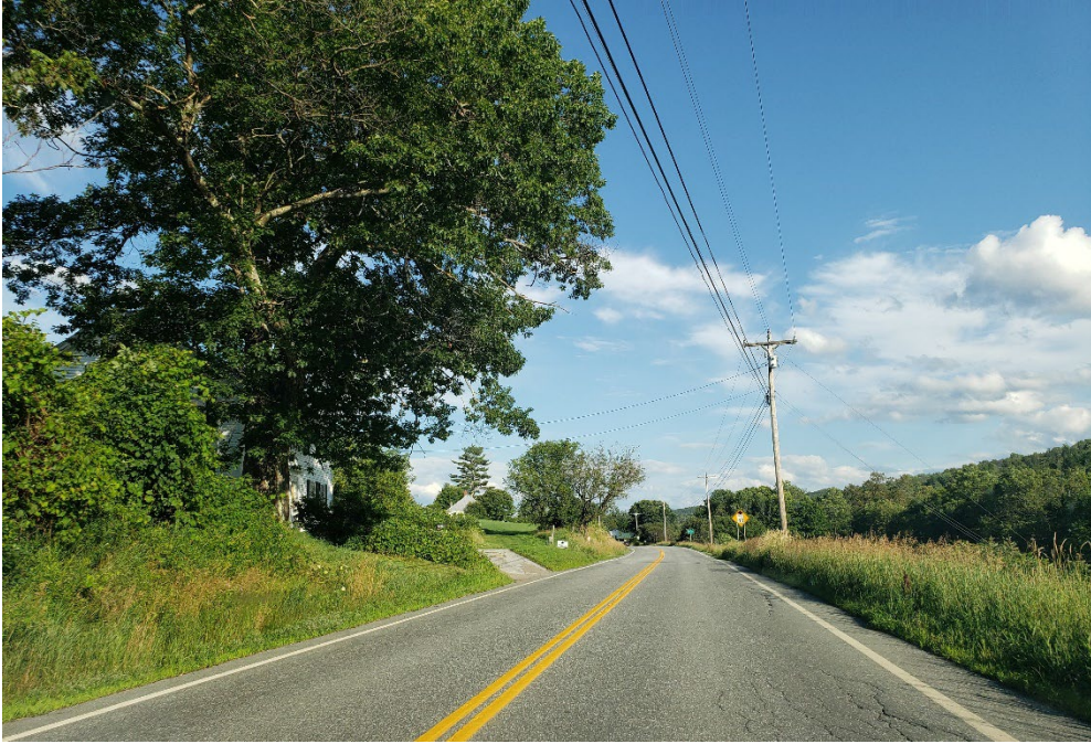
G: Northwestern Approach to Village (VT Route 25)
