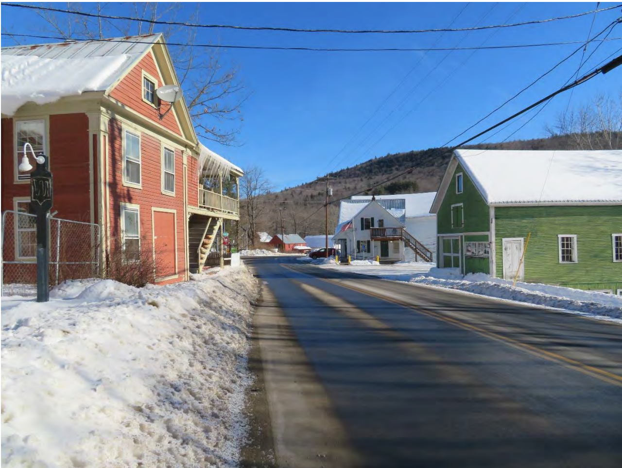
Photo#4: Route 100 at the edge of the Village Center at the Restaurant
