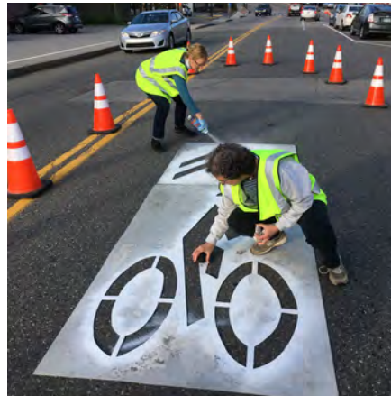
Top: Tactical Urbanism Materials and Design Guide workshop participants apply spray chalk with a homemade stencil in Fayetteville, AR (Street Plans). Bottom: In Burlington, VT (left) and Portsmouth, NH (right) volunteers use city-owned stencils to create bikeway markings with tempera paint and spray chalk (Street Plans). Each material and approach has its own strengths / weaknesses, as noted in the spec sheets that follow.
