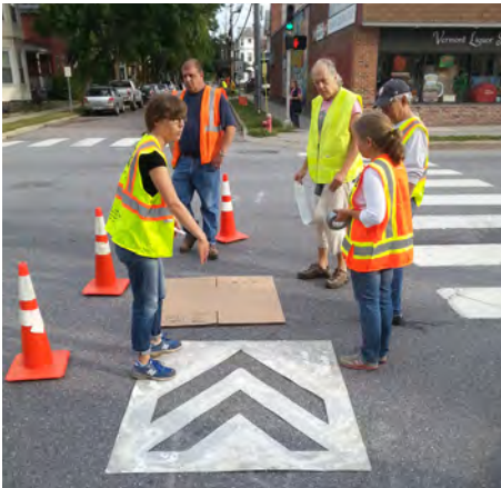
Top: Tactical Urbanism Materials and Design Guide workshop participants apply spray chalk with a homemade stencil in Fayetteville, AR (Street Plans). Bottom: In Burlington, VT (left) and Portsmouth, NH (right) volunteers use city-owned stencils to create bikeway markings with tempera paint and spray chalk (Street Plans). Each material and approach has its own strengths / weaknesses, as noted in the spec sheets that follow.
