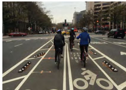
Hard plastic “armadillos” provide a low-lying and durable bike lane barrier. Left: Rogers, AR protected bikeway (Street Plans); Right: Washington, D.C. (Street Plans) Note: Washington D.C.’s Department of Transportation removed armadillos — spaced 15 ft. apart instead of 8 ft. or less. — because they failed to prevent u-turning in the bike lane as intended. They were replaced by the parking stops pictured above.
