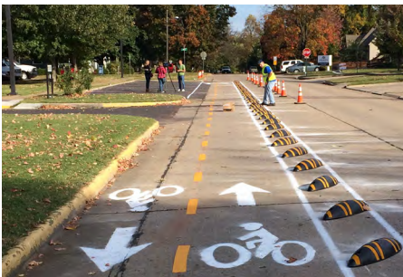
Hard plastic “armadillos” provide a low-lying and durable bike lane barrier. Left: Rogers, AR protected bikeway (Street Plans); Right: Washington, D.C. (Street Plans) Note: Washington D.C.’s Department of Transportation removed armadillos — spaced 15 ft. apart instead of 8 ft. or less. — because they failed to prevent u-turning in the bike lane as intended. They were replaced by the parking stops pictured above.
